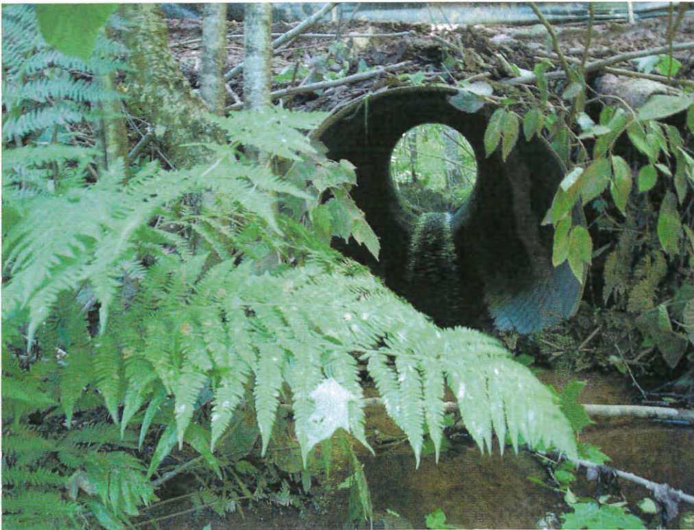
Existing 24-inch Diameter Culvert at Station 47+60 Inlet End
