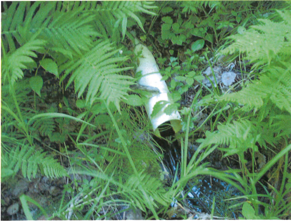
Existing 4-inch Diameter PVC Culvert at Station 44+80 Discharge End
