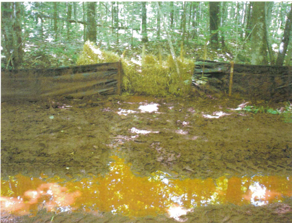
Hay Bale Dike at Station 12+62
