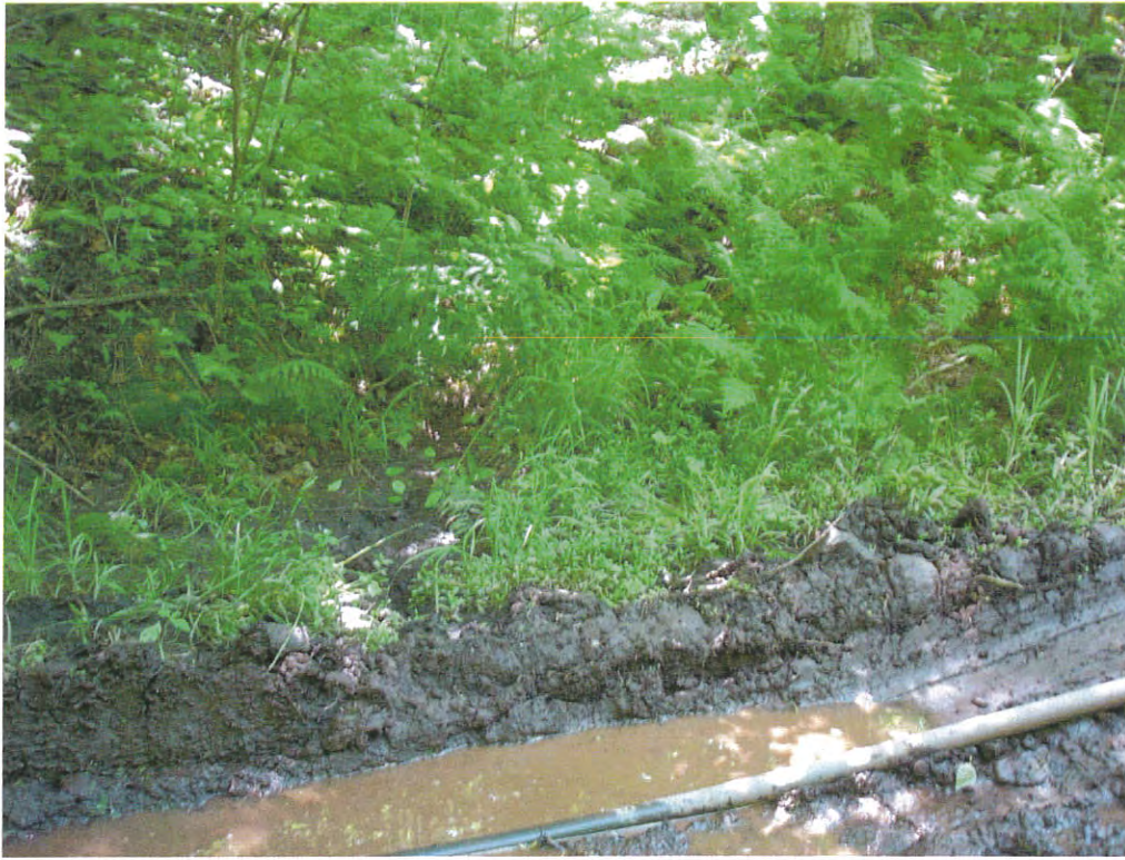
Proposed Culvert Location 42+80 Inlet View
