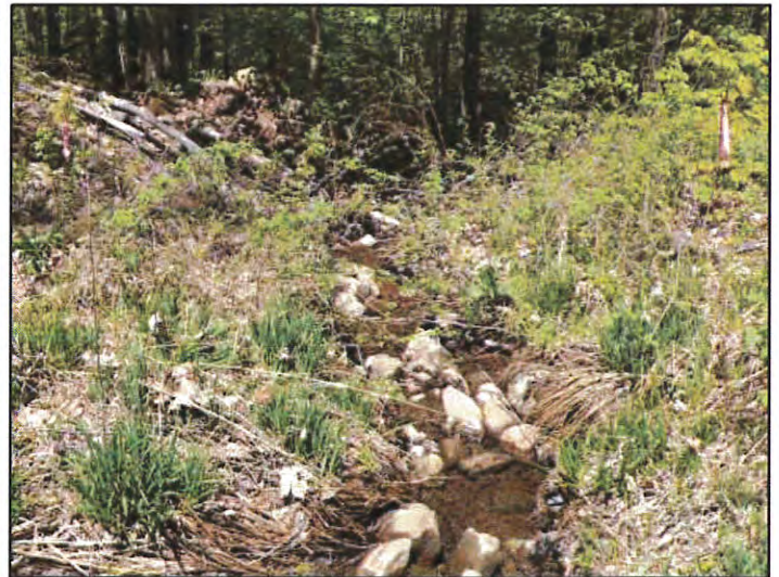
Drainageway in Wetland 8 - Looking North
