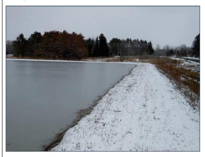
This photo of the infiltration basin in the Flambeau Mine industrial outlot was taken in Spring 2013, when the basin nearly overtopped and had to be pumped (Photo Credit: Wisconsin DNR, April 12, 2013).
