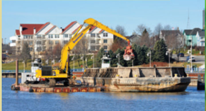
Contaminated sediment is dredged from the Sheboygan harbor.
