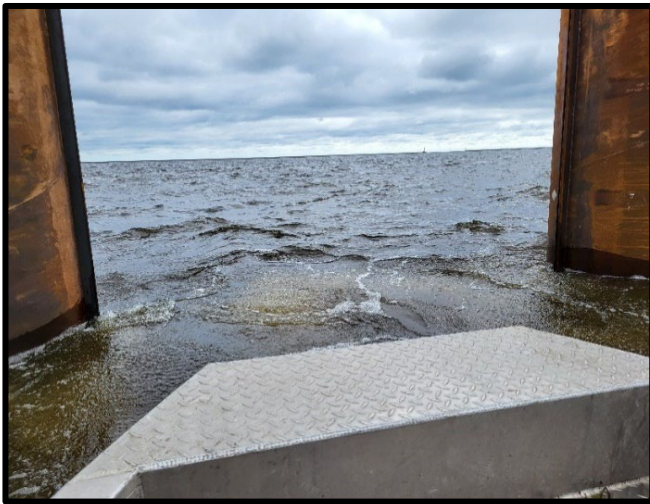
Image 4. (Left) DNR netting boat approaching the small opening in the wall of the DMMF to exit the facility. (Right) Close up image of the bubbles created by the bubble curtain intended to deter fish from entering the facility during the removal effort.
