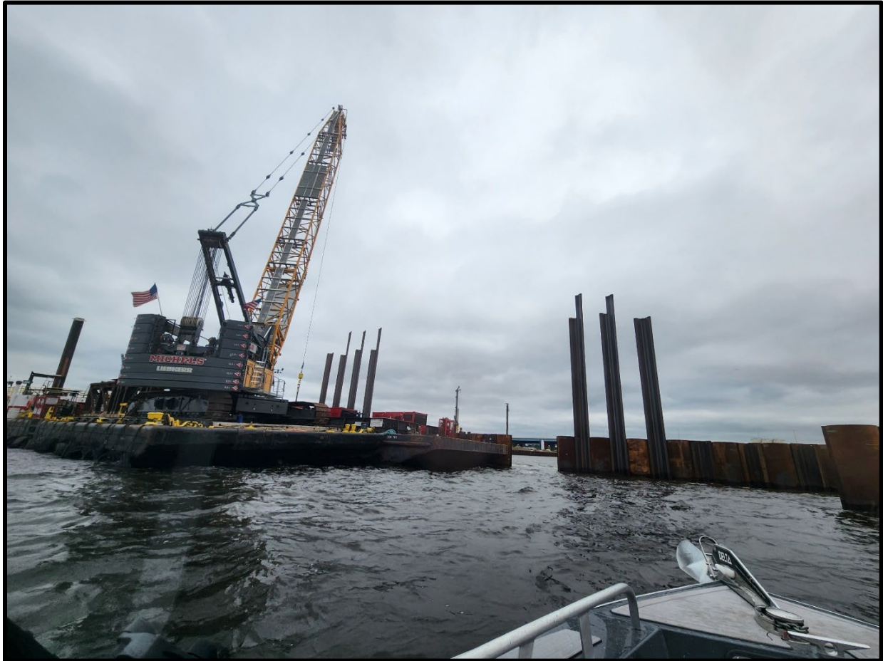
Image 10. A barge and crane working near the small opening in the wall of the DMMF.
