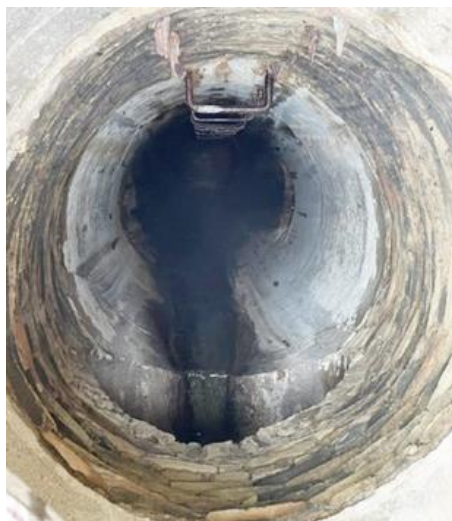
Figure 9. Manhole MH541D353 showing incoming dry weather flow.
