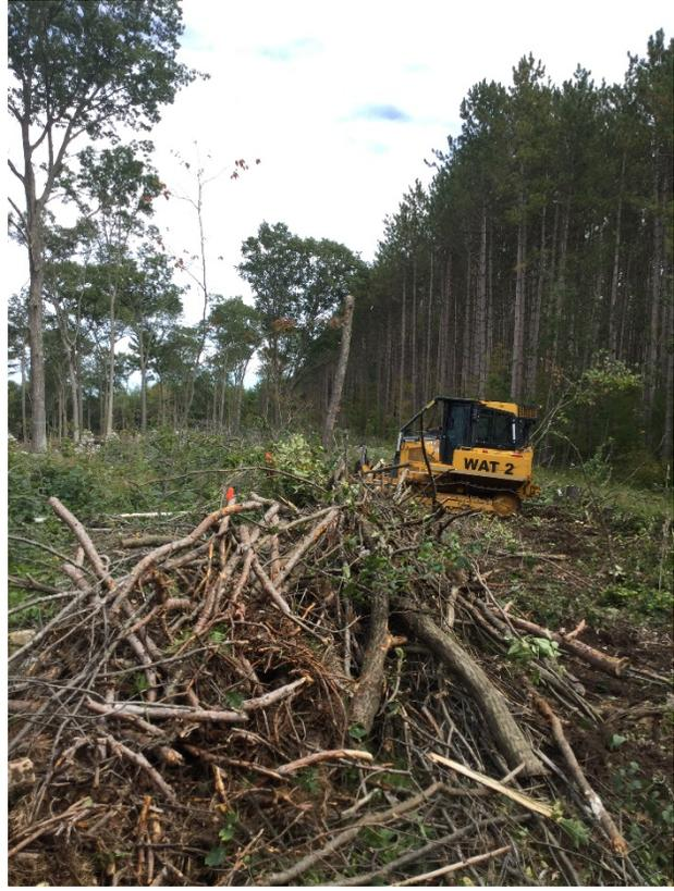
*Figure 12 Process of constructing a slash wall.*
