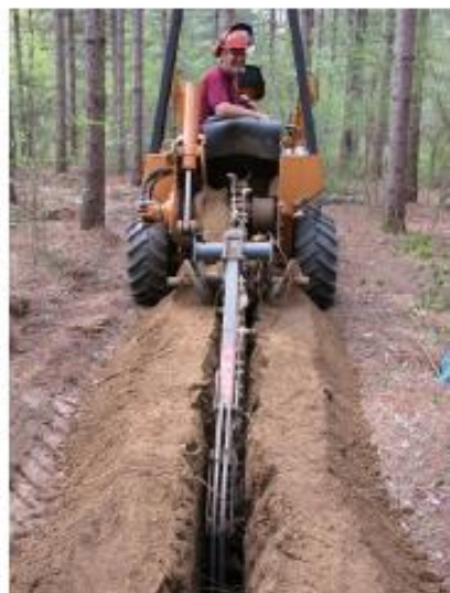
Roots are severed using a trencher
