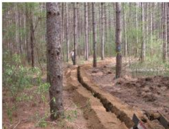
Right after the site is trenched.
