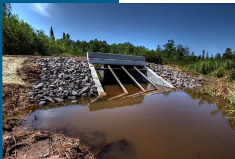
The upgraded Nicoletti Road culvert, shortly after installation (August 2015).
