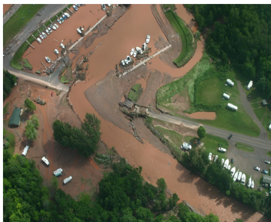
Saxon Harbor, Iron County After July, 2016
