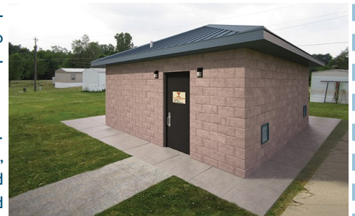
Tornado Safe Room
