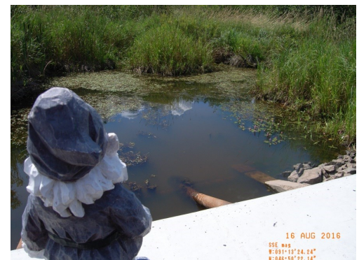
The Nicoletti Road Gnome faithfully watches over the upgraded culvert.
