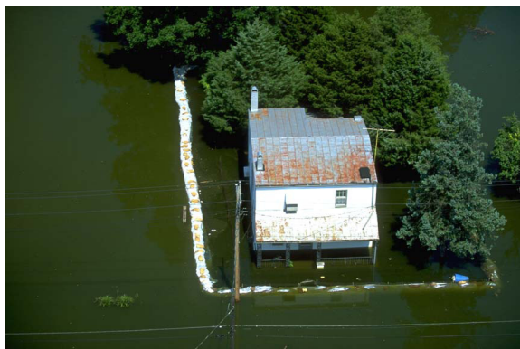
-Flooded residential septic system
