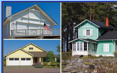
Wind Retrofit Guide for Residential Buildings
