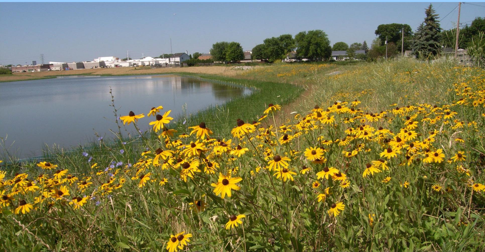
**Detention/retention ponds can store storm water runoff, decreasing flash flooding in urban areas.**
