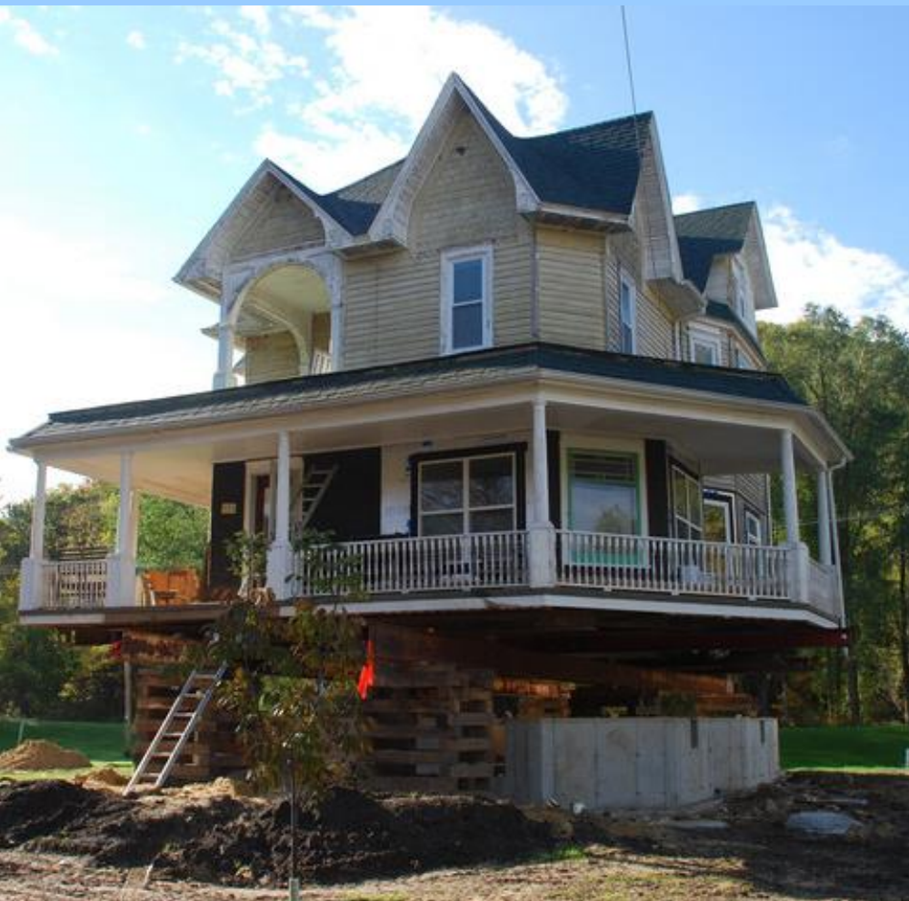
Elevation raises a structure out of the floodplain.
