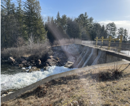
Downstream view of the outlet dam on Chute Pond. Photo credit T. Paoli.
