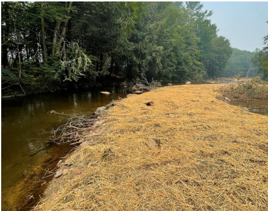
Picture 1 Eleven points bars were added to the stream. They were mulched and seeded upon their completion.
