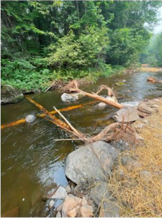
Picture 2 and 3 Rocks, root wads and wood structures were added to the stream as habitat structures.
