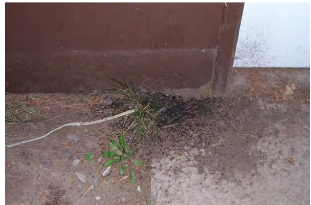
Bat guano in front of garage
