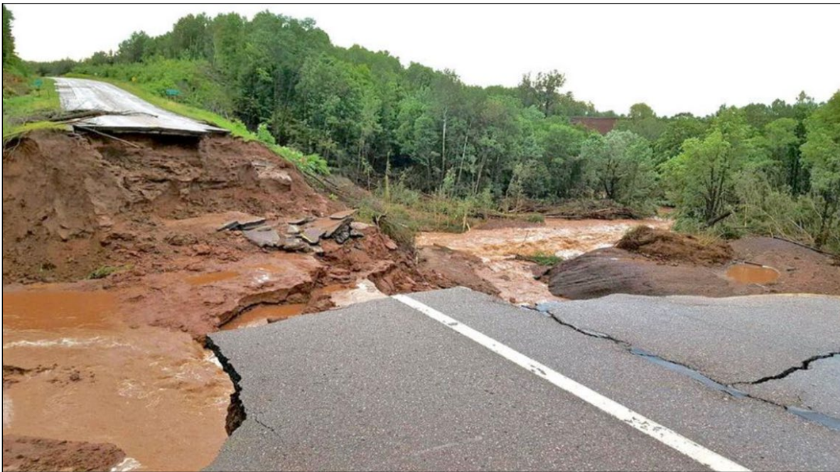
Figure 5.6-19 Valley Landslide and Washout of Highway 13 at Silver Creek, July 2016. Photo: Ashland County Land and Water Conservation Department
