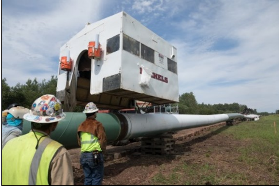
Figure 2.6-6 Pipe welding. Photo: Enbridge
