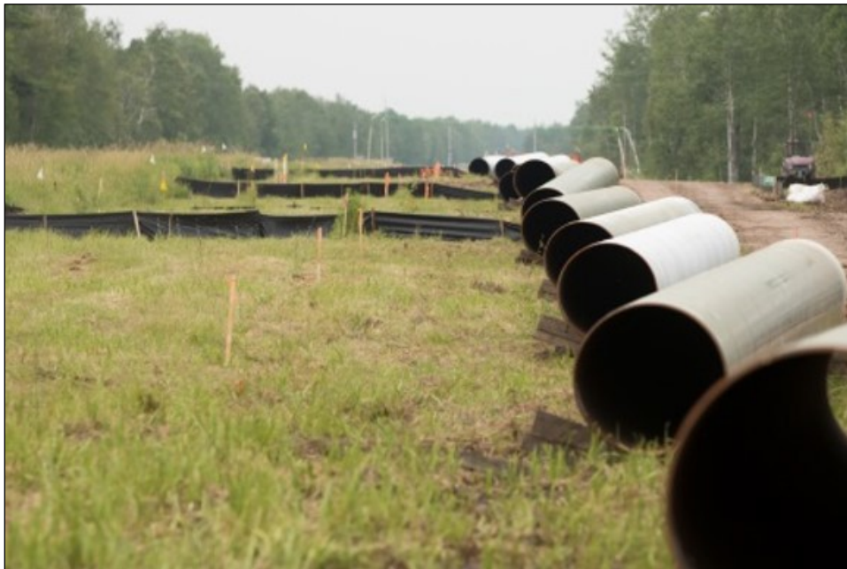
Figure 2.6-2 Example of pipe stringing. Photo: Enbridge
