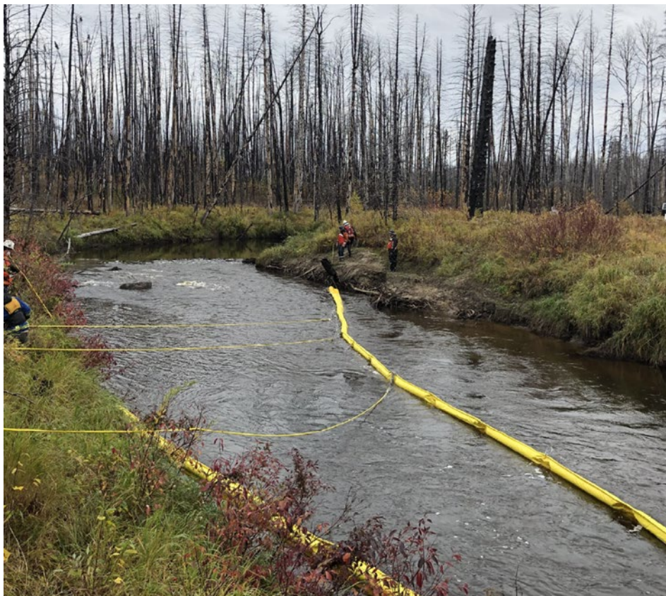
Figure 6.3-9 Deployment of a containment boom in a river. Source: RPS Operations Assessment: Oil Spill Report; Appendix AH
