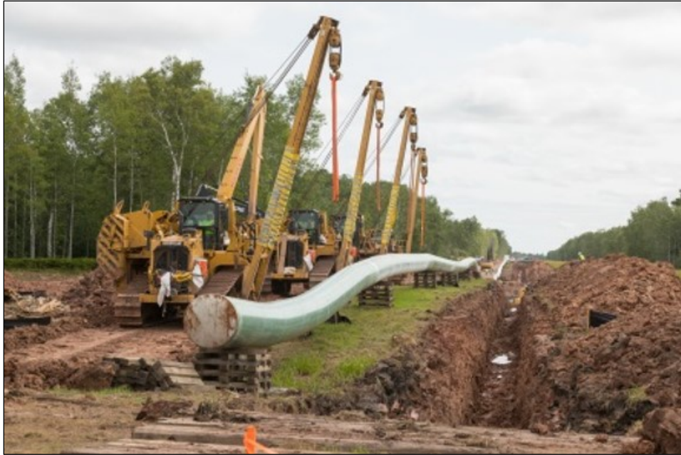
Figure 2.6-7 Sideboom tractors lowering pipe into a trench.
