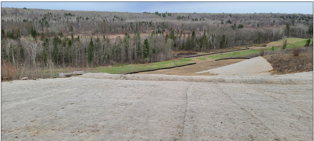
Figure 2.6-9 Slope breakers. Photo: Enbridge
