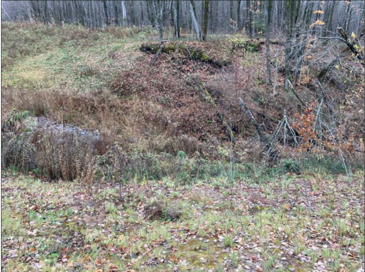
Figure 5.6-23 Newly formed gully along Potato River Road with riprap stabilization, October 2023. Photo: Samuel Hermanstorfer, DNR
