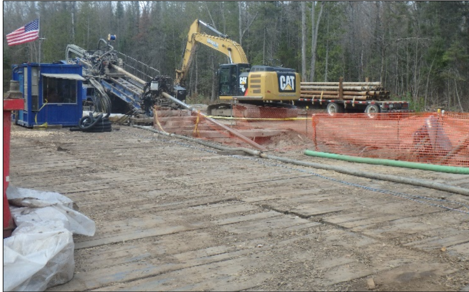
Figure 2.5-4 HDD drill rig.
