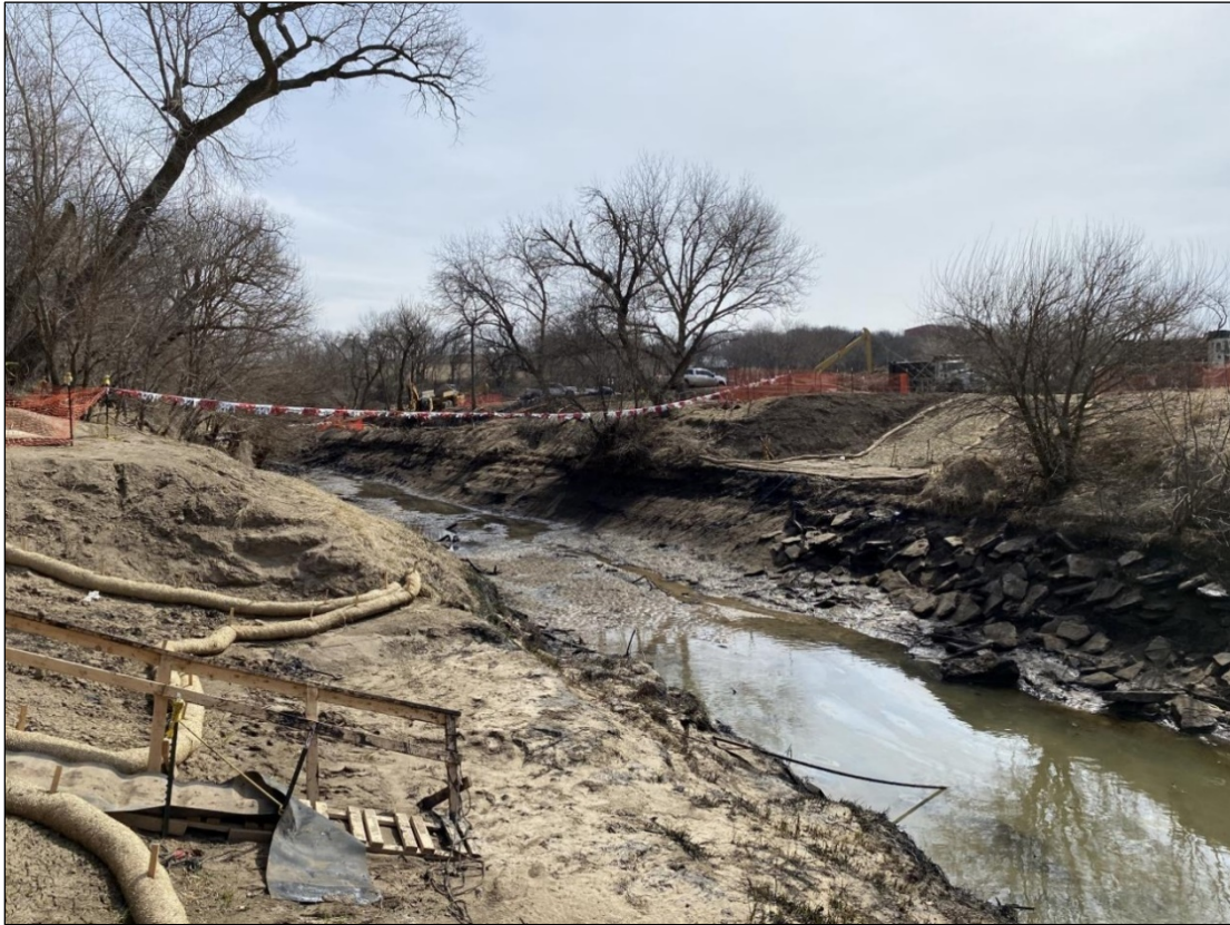
Figure 6.4-23 Dewatered section of Mill Creek
