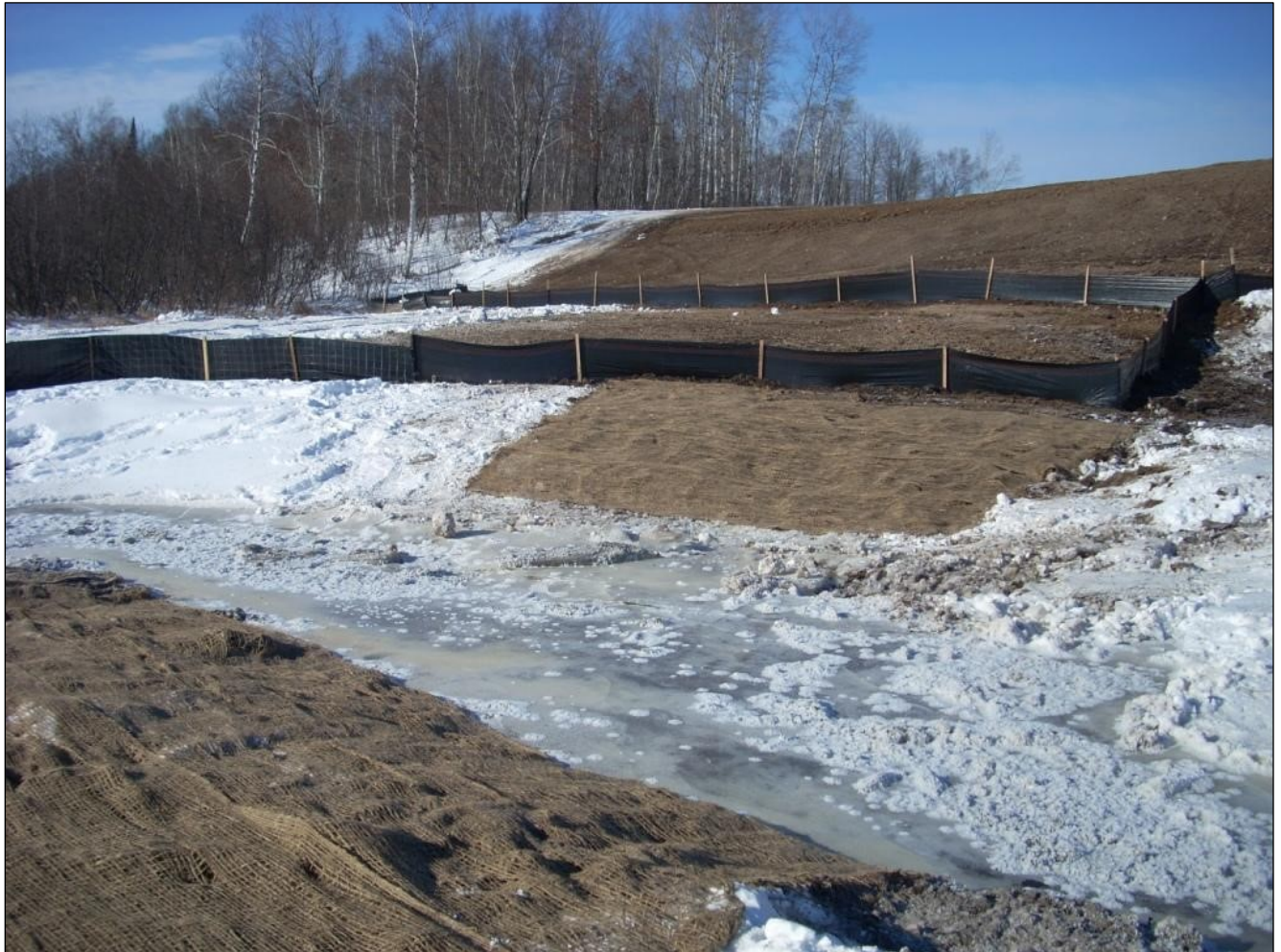
Figure 5.6-10 Erosion control measures along a riverbank during winter conditions.
