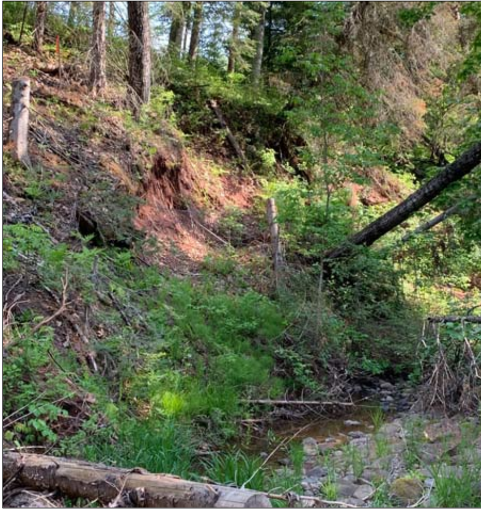
Figure 2.1-8 Example of a slope failure due to erosion.
