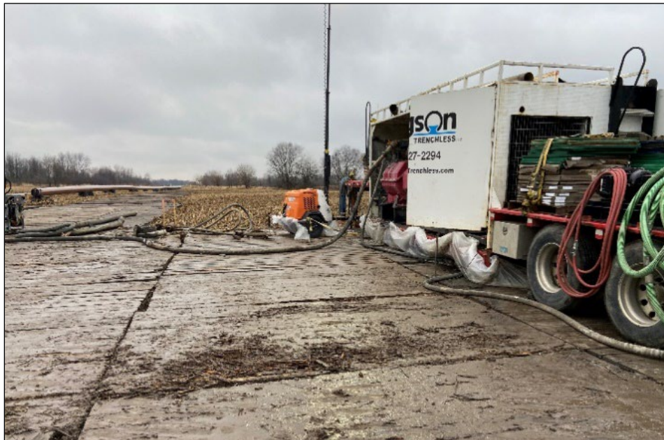
Figure 2.5-5 HDD exit side with pipe.
