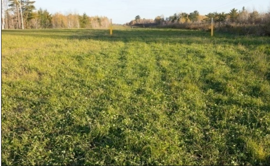
Figure 2.6-8 Revegetated pipeline ROW. Photo: Enbridge
