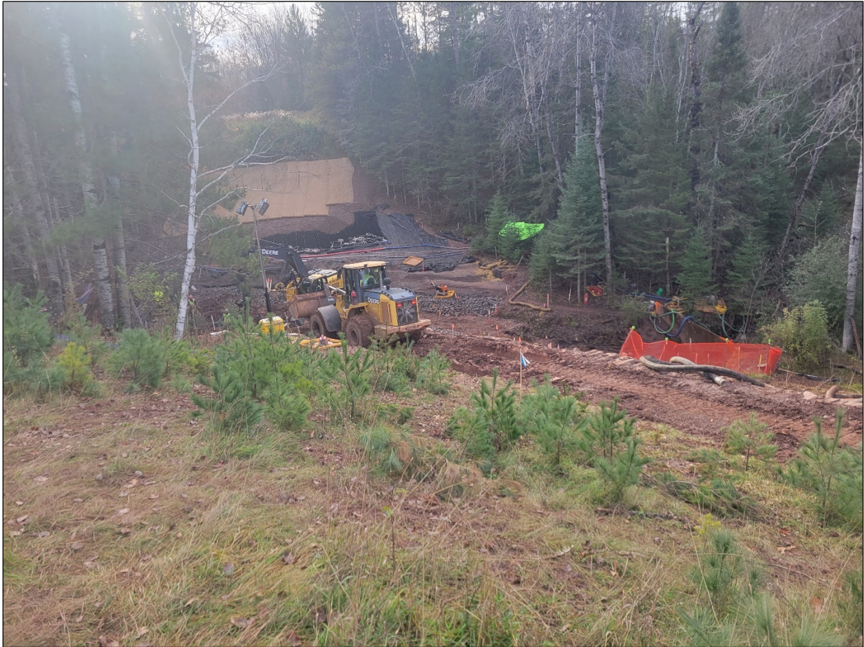
Figure 5.6-28 Enbridge’s Slope 20 restoration project (2024), in progress.
