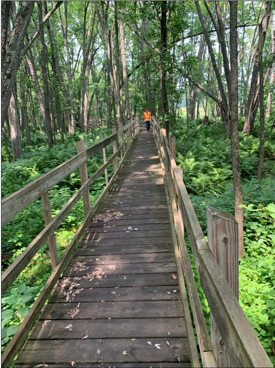
Figure 5.12-3 Boardwalk at North Country National Scenic Trail. Photo: Dreux J. Watermolen, DNR
