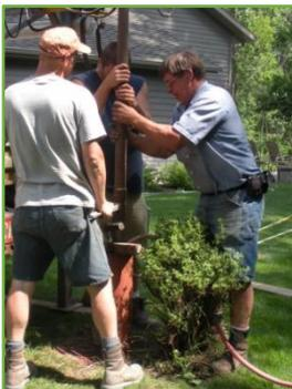
**Air vacuuming** is an option where an airline is attached near the bottom of a 2 to 4-inch diameter steel pipe that is lowered in the well. The air exits up the pipe. The flow creates suction and vacuums up debris a few feet below the pipe.
