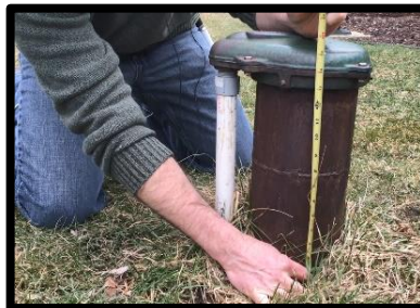
Well height – current code 12-inch minimum
