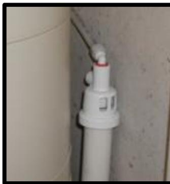
Manufactured air gap for water treatment backwash
