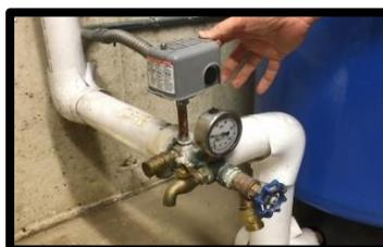
Well pump pressure switch box, pressure gauge and source sample faucet
