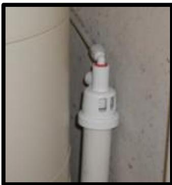
Manufactured air gap for water treatment backwash
