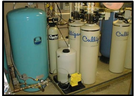
Chlorination injection system and pre-treatment devices
