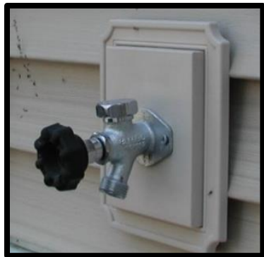
Faucet with built-in vacuum breaker
