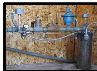
Above ground discharge & controls on discharge line
