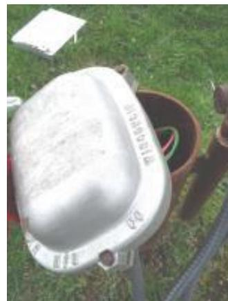
Open cap, warped gasket, broken conduit    Gasket sticking out, loose bolt    Well cap can be pulled off
