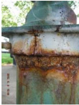
Cracked pump base, corroded
