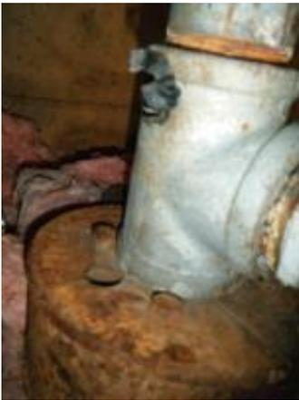
Missing bolt, corroded
