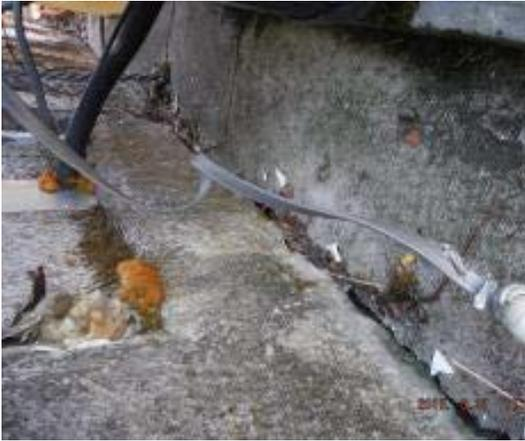
Pump wires not completely enclosed
