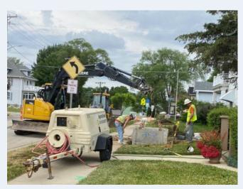
A Stoughton crew replaces a lead service line. The city successfully used directional drilling for most LSL replacements and only dug open trenches in situations where other methods were not feasible.
