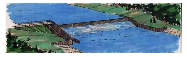
**Gravity Dam with Stoplog Spillway**
