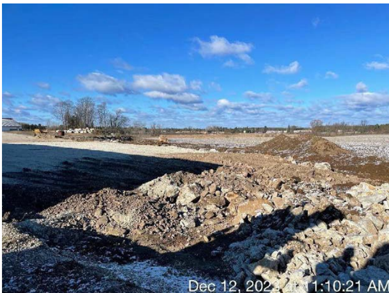
Photo 43. The north side of the feed storage area, where excavation was done. Bedrock was blasted and excavated from the site. This photo was taken facing northwest.
