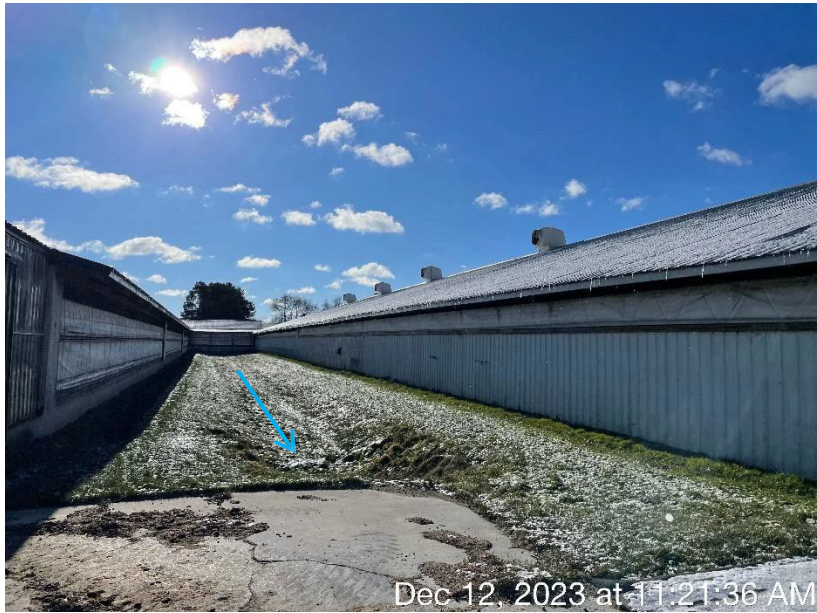
Photo 63. The outlet that discharges stormwater from the grassed swale pictured in Photo 62. The outlet is covered by the concrete slabs.
