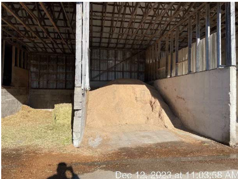
Photo 60. Commodity storage bays at Gilbert Farms.
