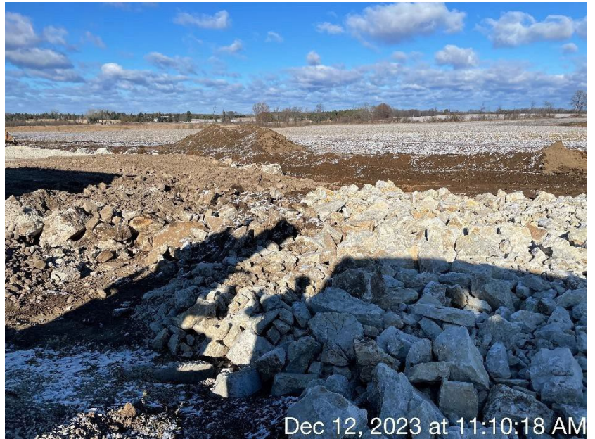
Photo 43. The north side of the feed storage area, where excavation was done. Bedrock was blasted and excavated from the site. This photo was taken facing northwest.
