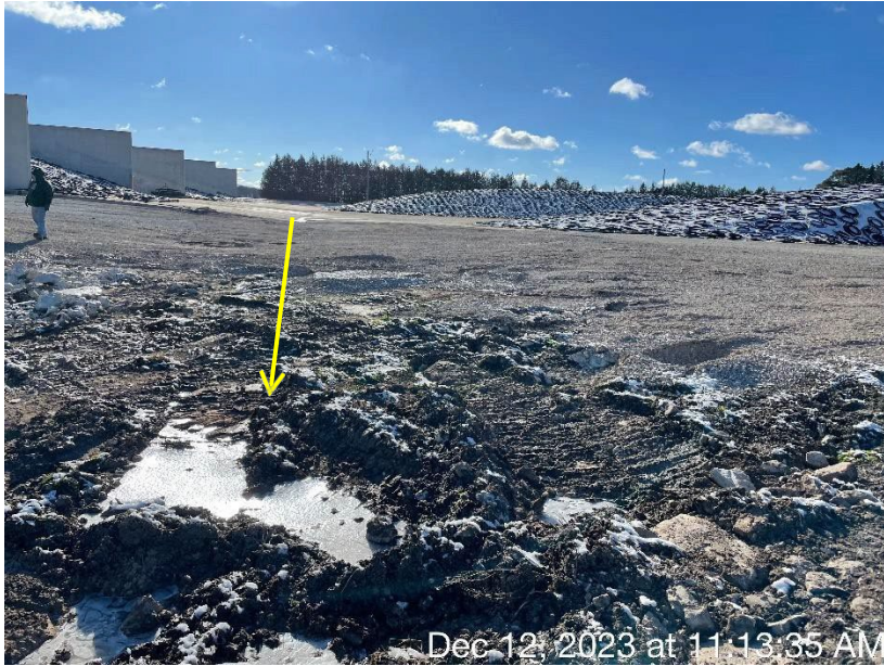
Photo 54. The flow path of runoff from the north side of the feed storage area. The yellow arrows represent the flow path.
