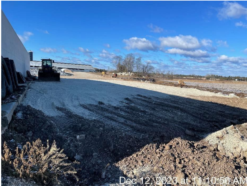
Photo 45. The north side of the feed storage area, where excavation was done. Bedrock was blasted and excavated from the site. This photo was taken facing west.
