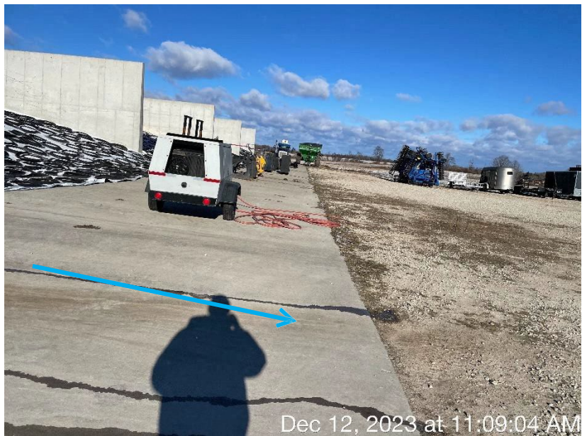
Photo 40. The east side of the feed storage area, which is sloped to convey stormwater away from the feed storage area.
