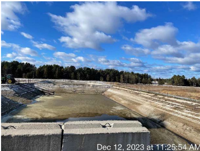
Photo 9. WSF 1 at Gilbert Farms, which accepts manure from the freestall barns. WSF 1 is located on the northwest corner of the production site. The photo was taken facing west.
