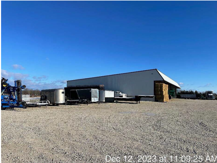
Photo 67. The machine shed and parking area located east of the feed storage area.
