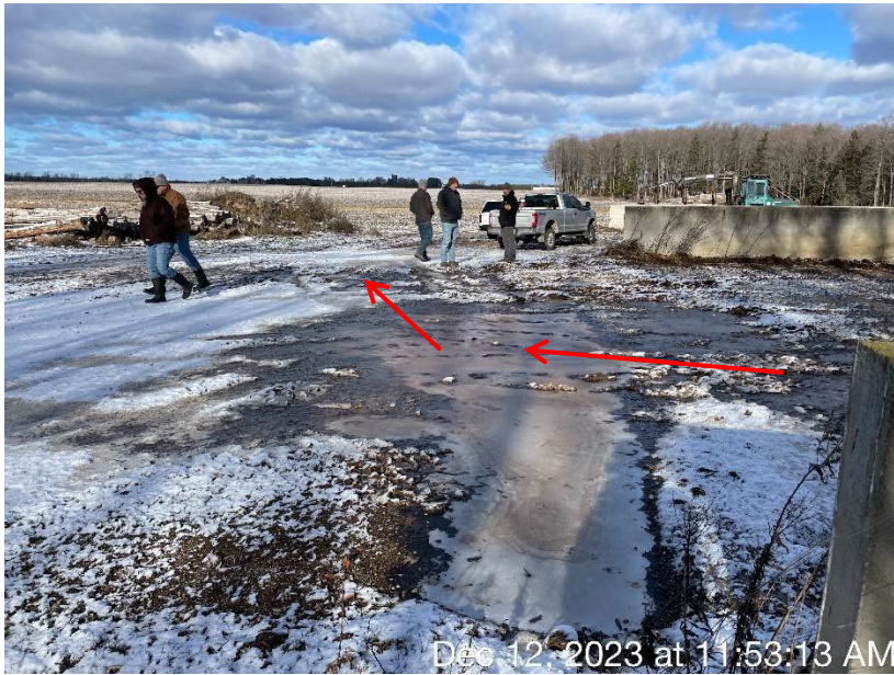
Photo 23. The flow path of runoff from the satellite stacking pad, represented by the red arrows. There are no runoff controls currently in-place.
