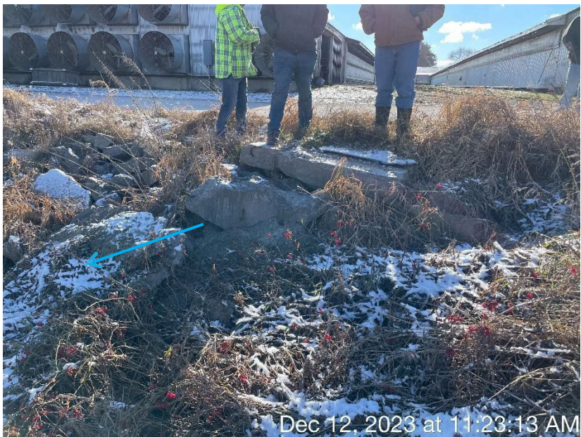
Photo 63. The outlet that discharges stormwater from the grassed swale pictured in Photo 62. The outlet is covered by the concrete slabs.
