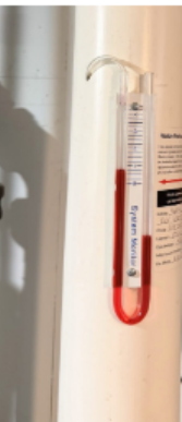
Example of vacuum gauge mounted to the interior wall.
