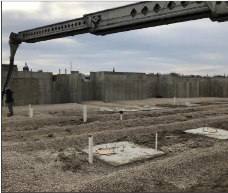
Sub-Grade Pipes
