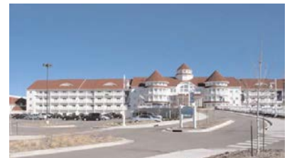
Blue Harbor Hotel anchors mixed use development
