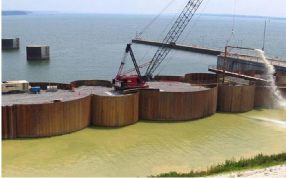
Construction of the Kentucky cellular cofferdam (C. J. Mahan Co., 2017).
