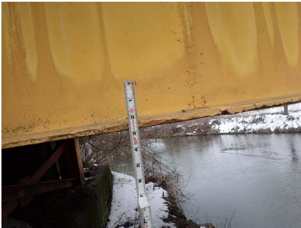
View of typical painted over corrosion on girder, looking north.
