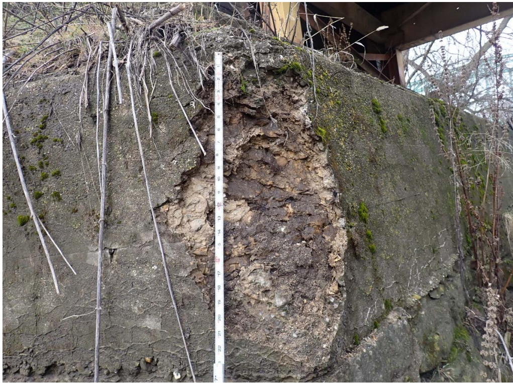
View of typical spalling on concrete abutment cap, looking west.
