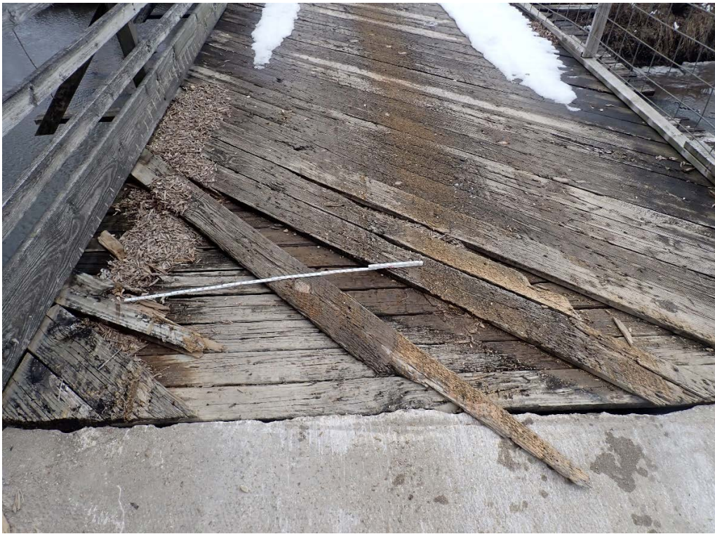
View of missing boards at west end of deck, looking east.
