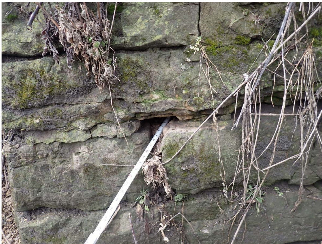
View of typical loss of mortar on masonry abutment, looking west.
