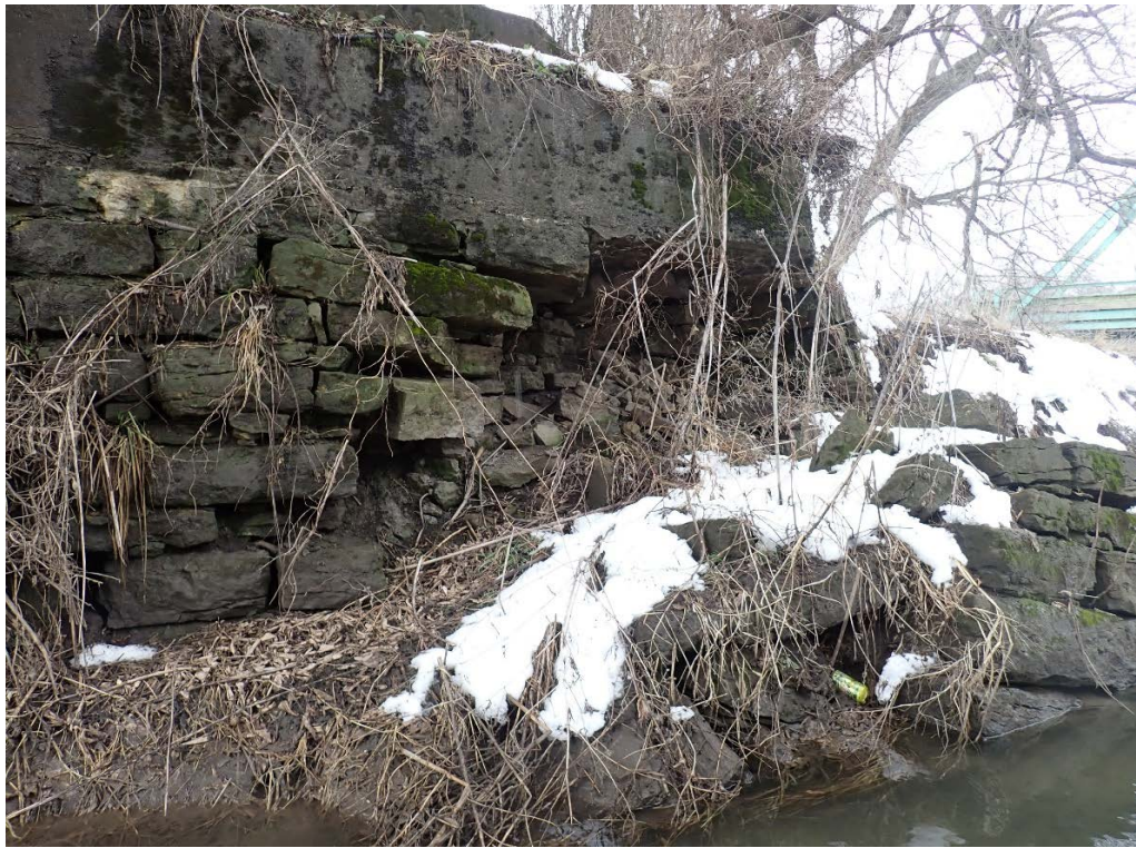
View of masonry failure at northwest corner of west abutment, looking west.
