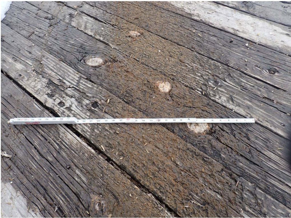
View of typical snowmobile wear, looking east.
