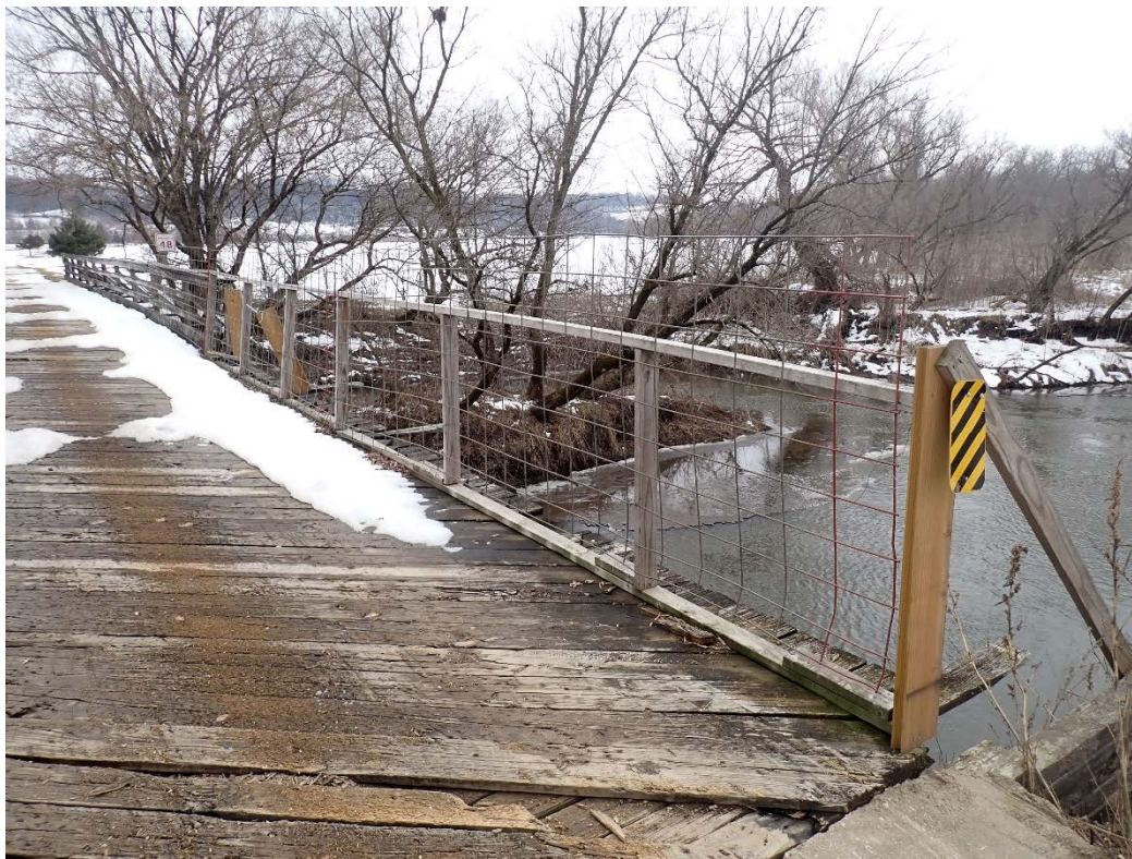
View of southwest railing missing/temporary repair, looking east.
