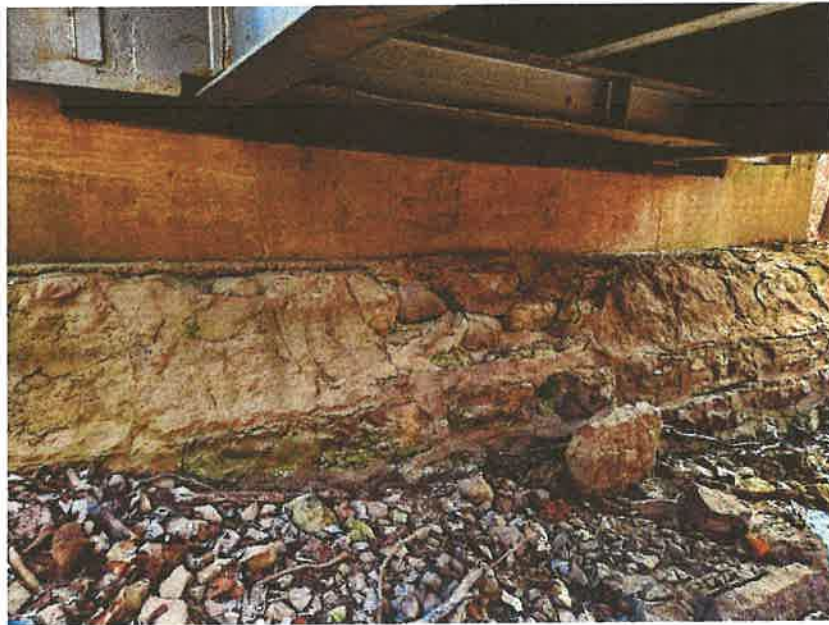
VIEW OF ABUTMENT AND UNDERSIDE OF SUPERSTRUCTURE
