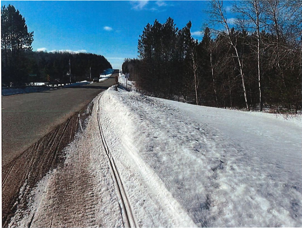
North of Bridge Looking South
