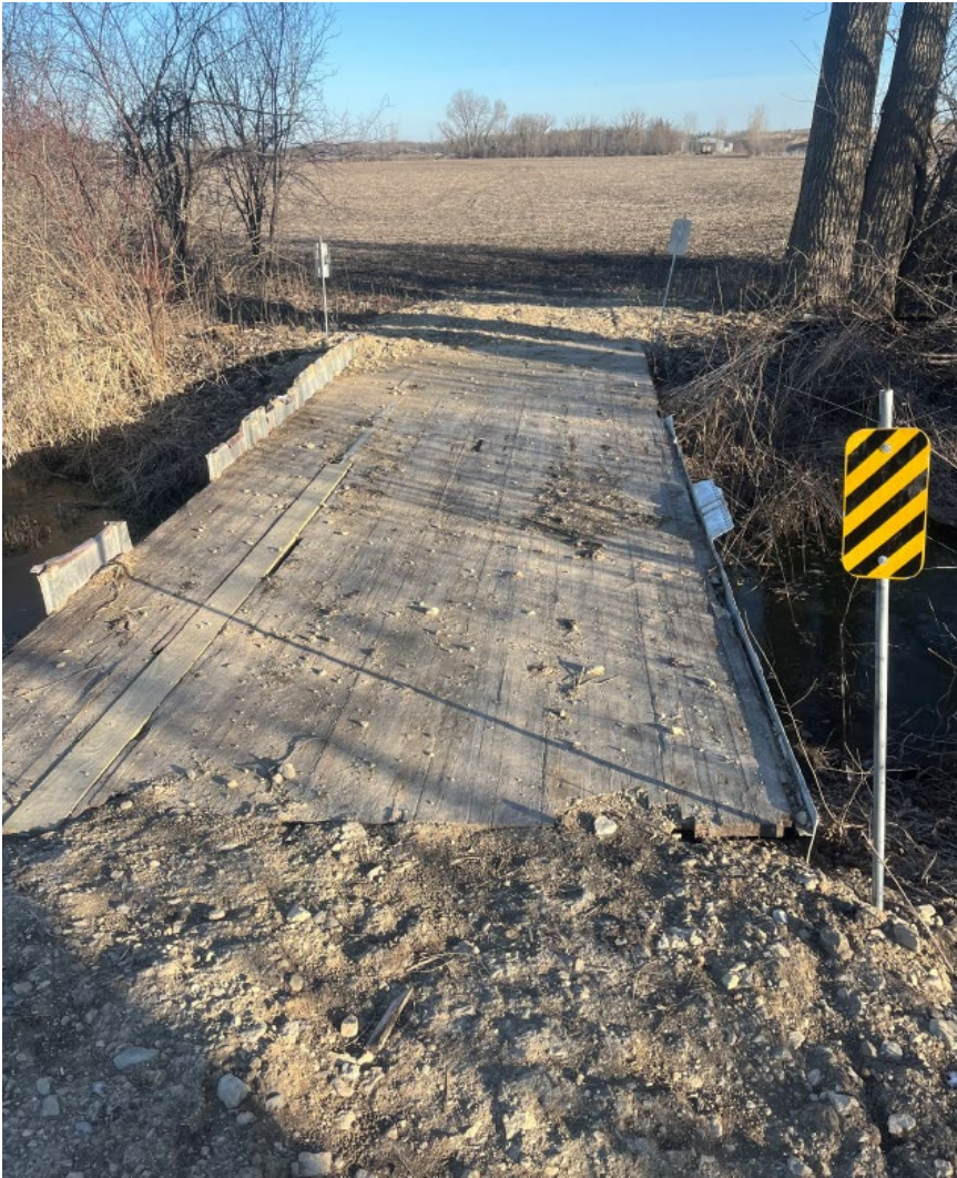
Temporary Bridge Currently In Place
