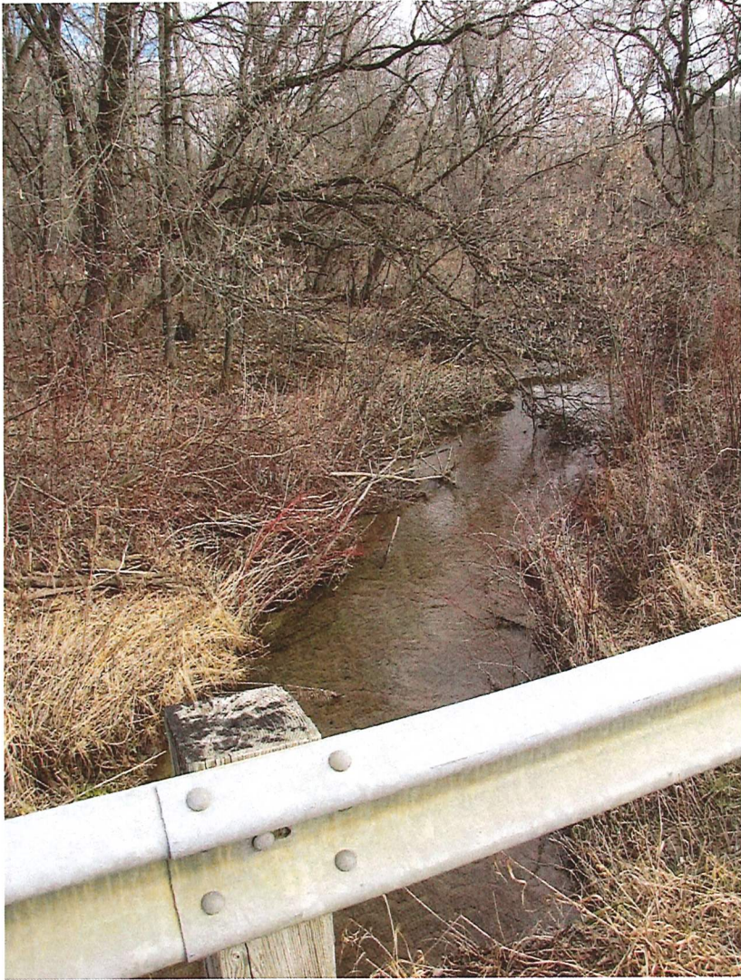
Middle Bridge. Upstream view. (I was facing west.)
