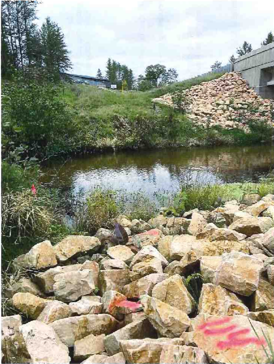
Illustrates "flat bottom" ditches installed by WisDOT
