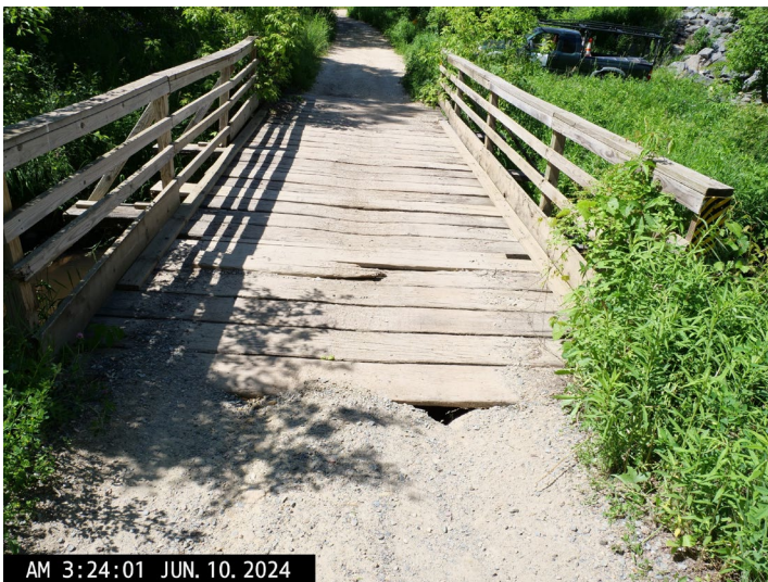
South End of Deck looking to North
