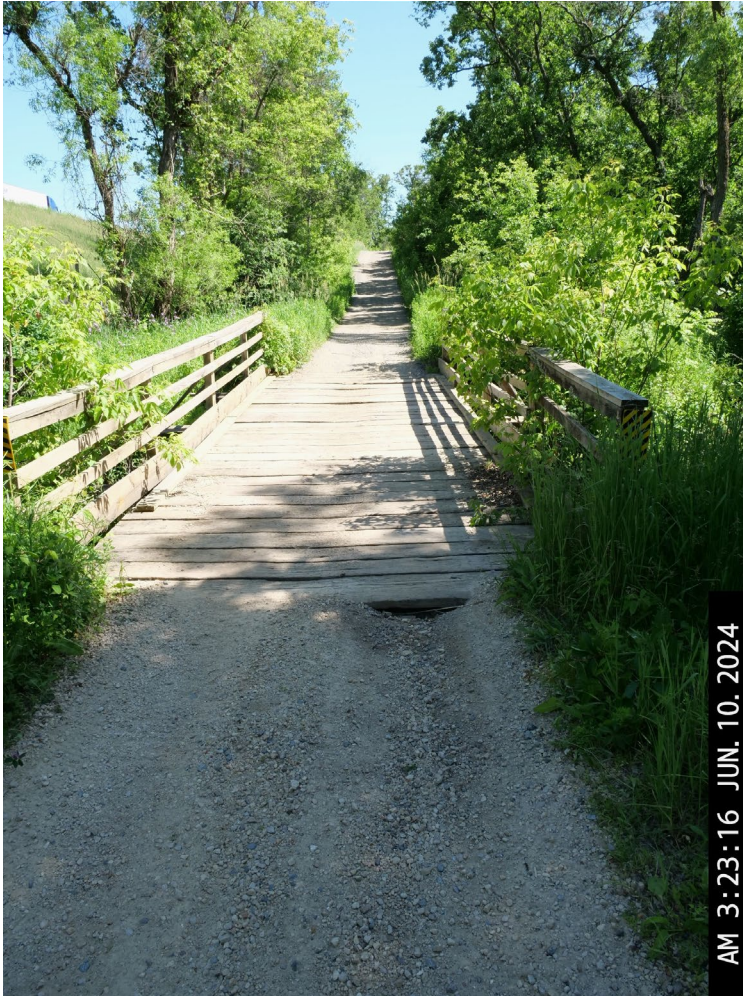
North End of Deck looking to South
