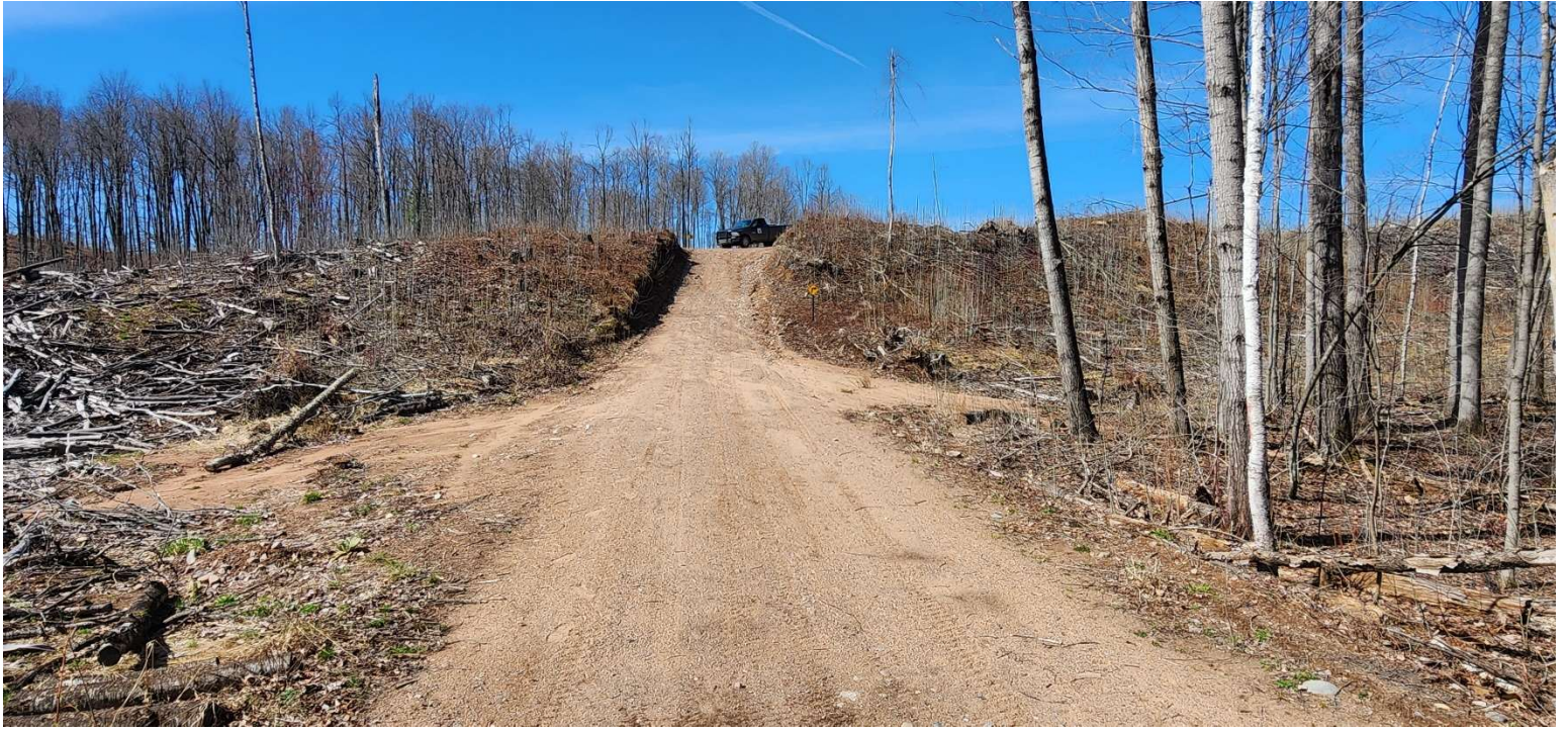
Hill 5: Washout erosion
