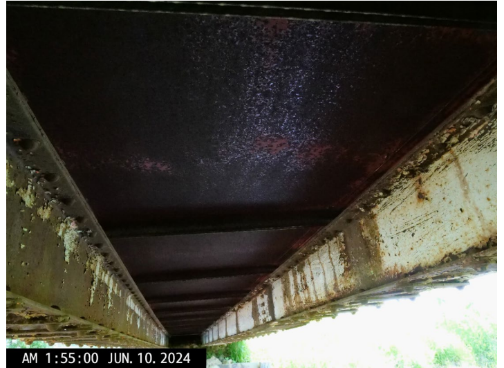
Typical Bottom of Diamond Steel Tread Plate Deck
