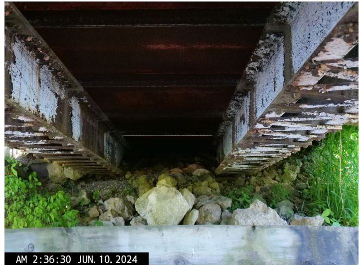
South Abutment Close Up
