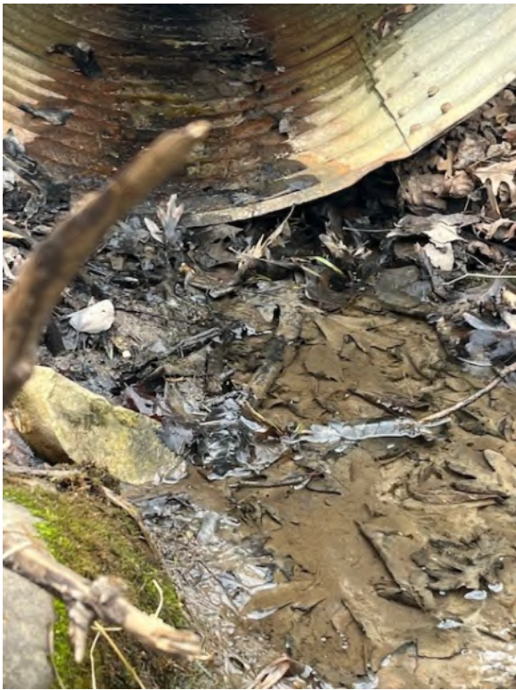
Water is flowing around and under the culvert and undermining the above trail.
