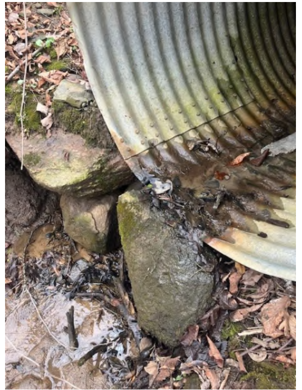
Water is flowing around and under the culvert and undermining the above trail.
