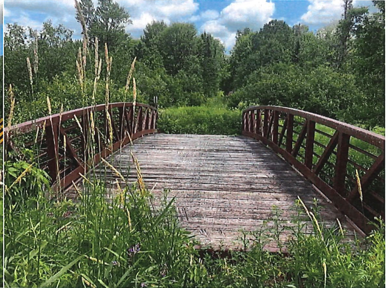
Bridge Deck Looking East
