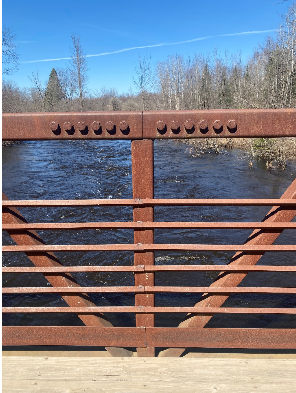
Bridge center connection. Looking upstream.
