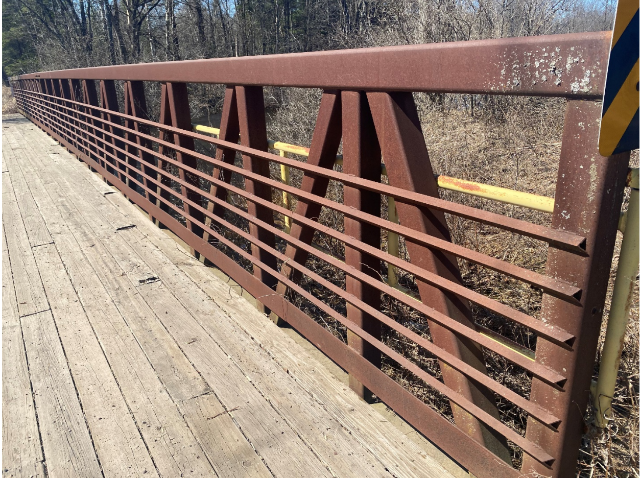
Looking west from east approach at inside of upstream railing.
