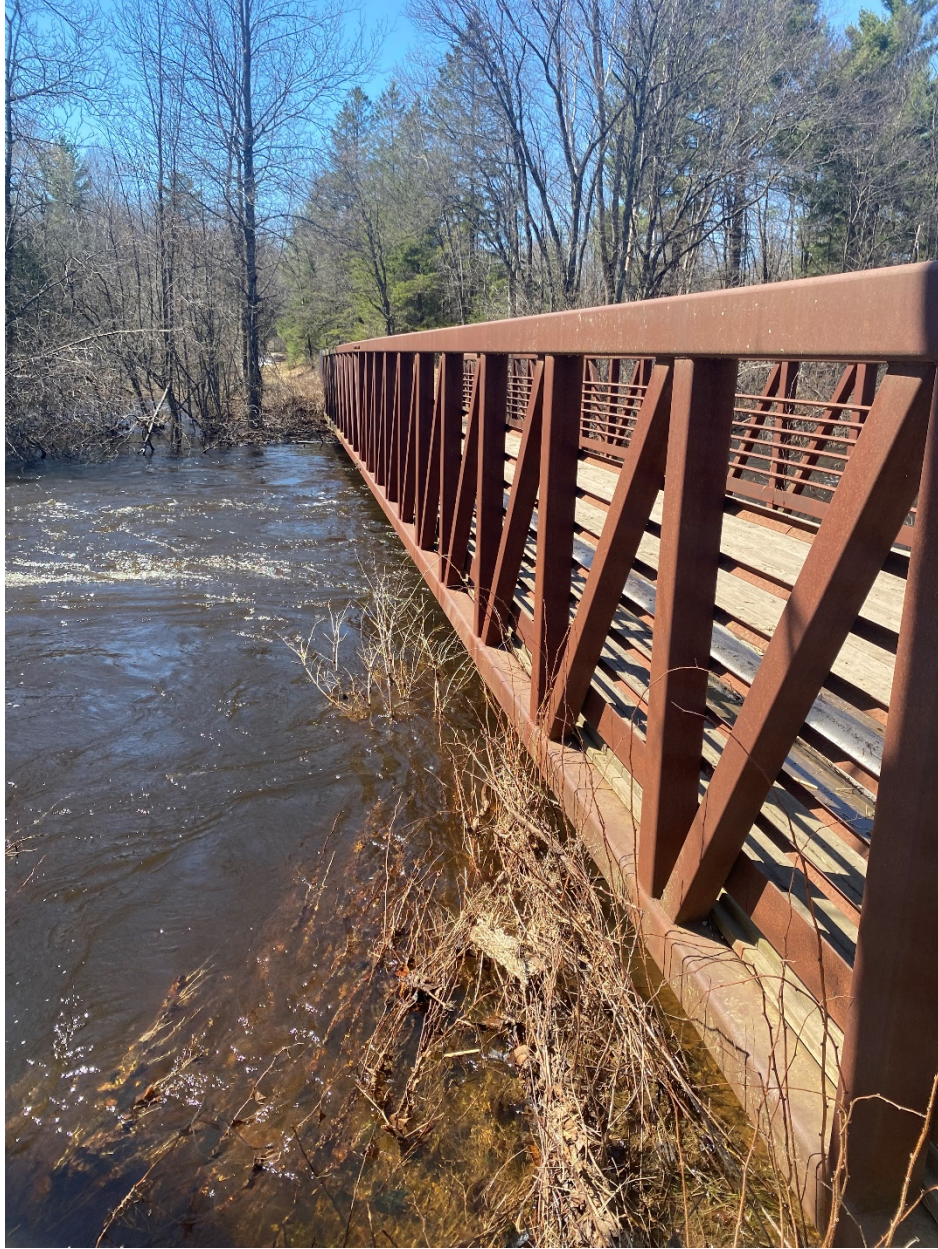
Looking west at the outside of the downstream railing.
