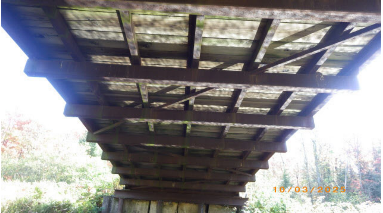
Typical deck underside
