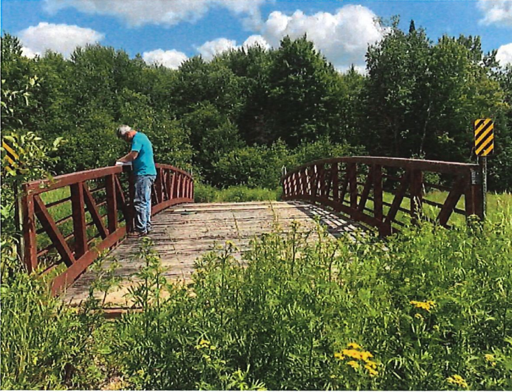
Bridge Deck Looking West
