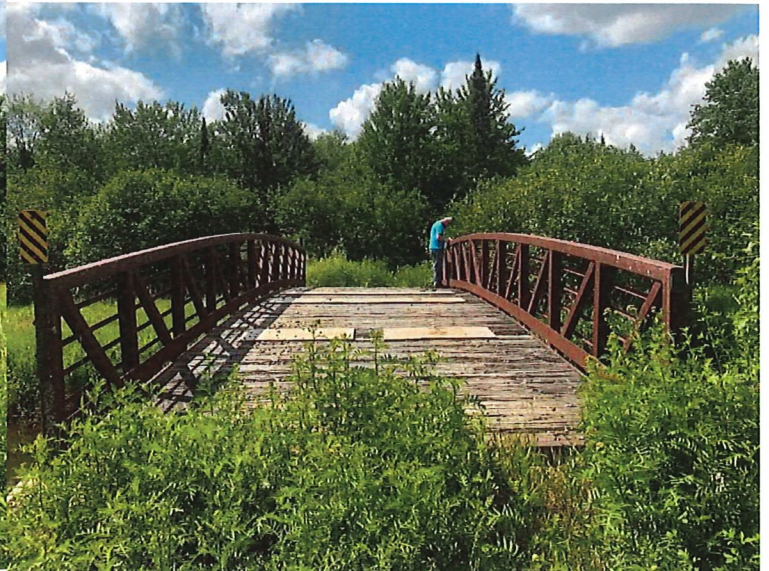
Bridge Deck Looking East
