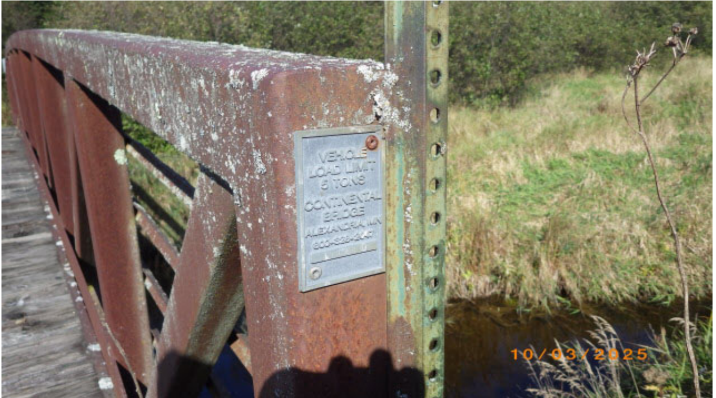
Continental Bridge placard, 5T load limit
