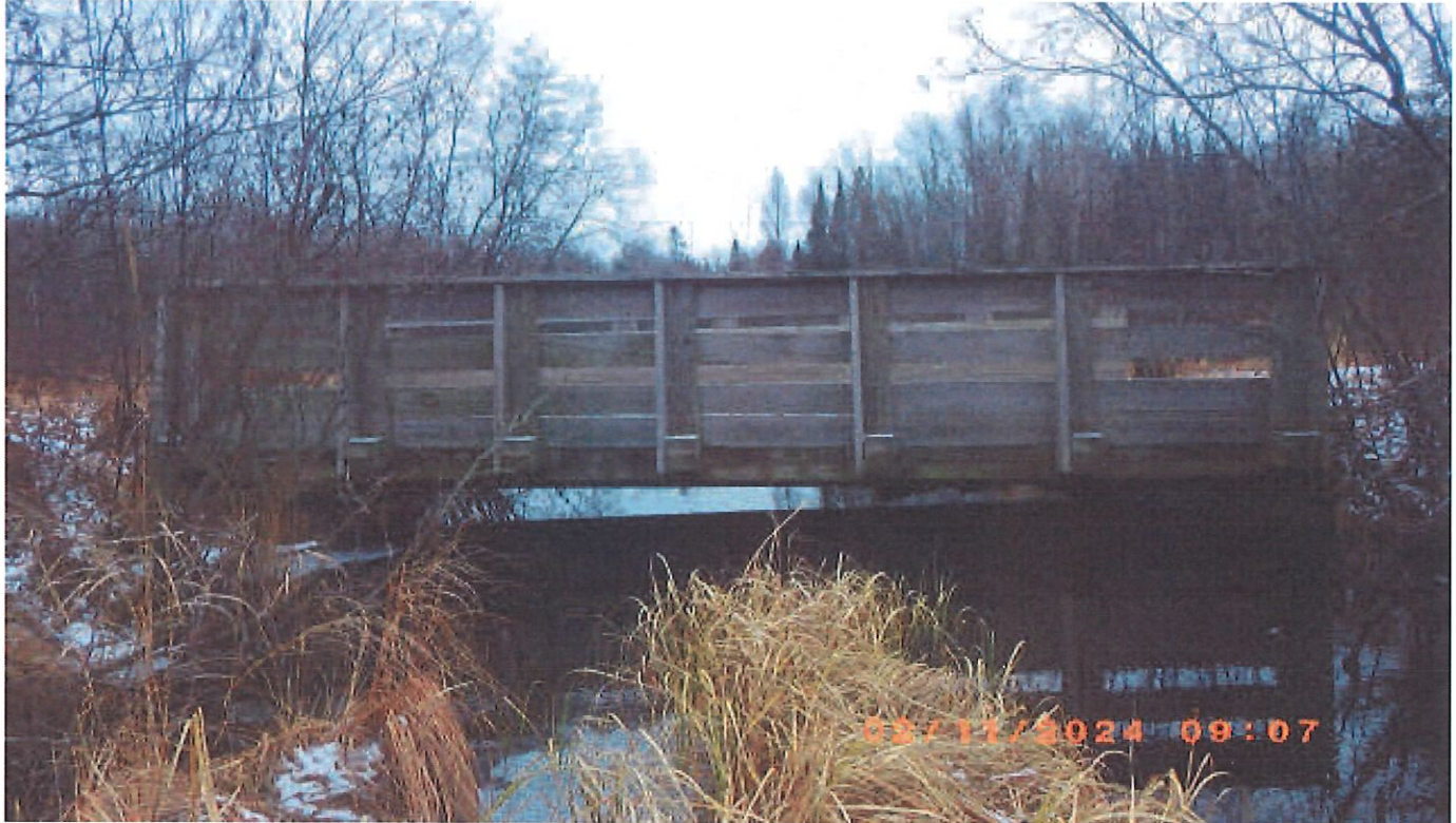
Elevation view from upstream
