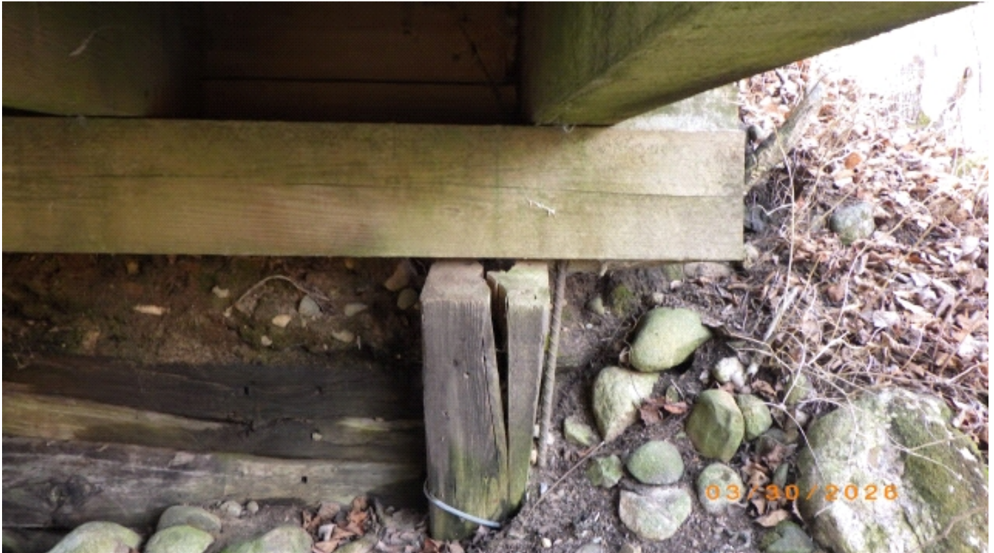
West end of South Abutment.
