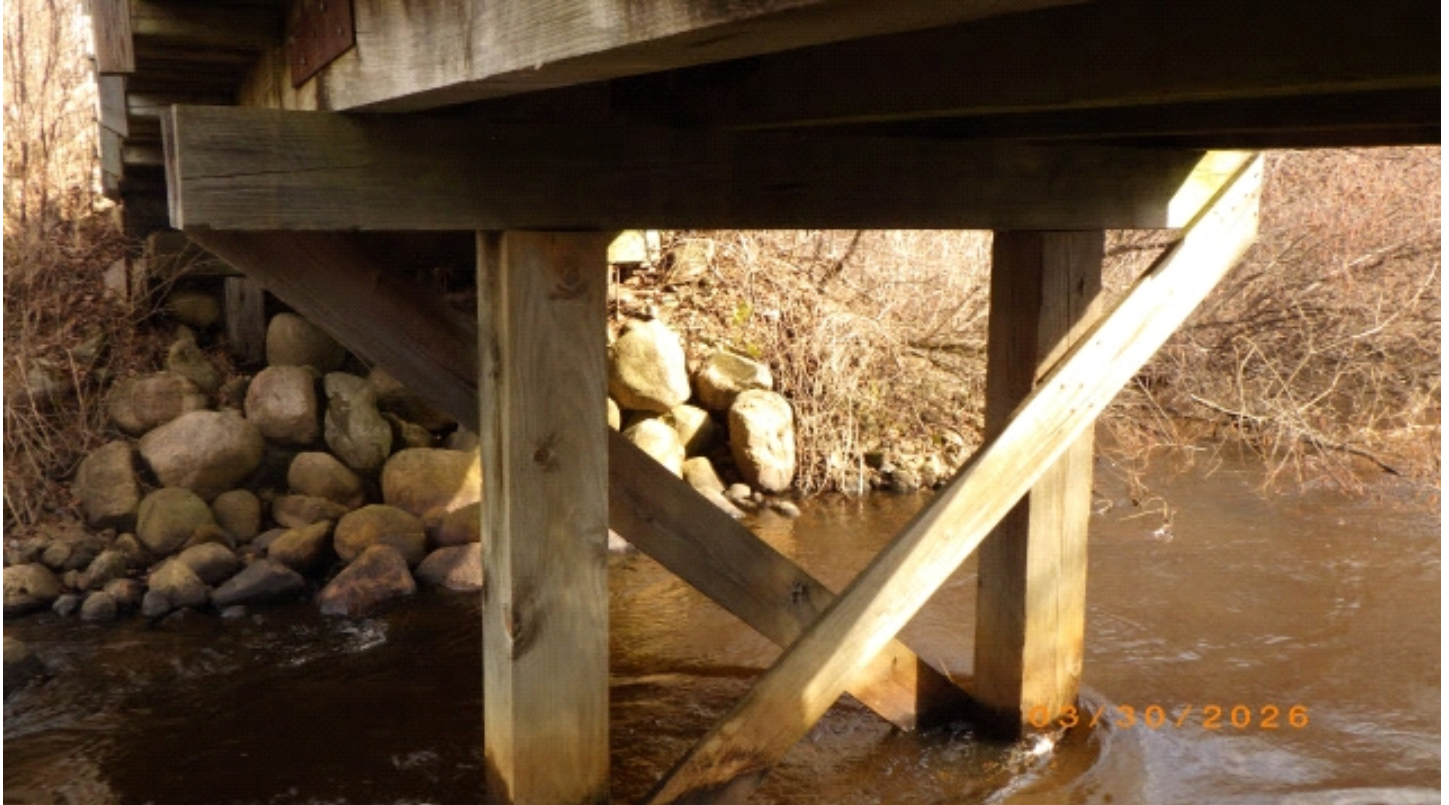
Looking at pier, North.
