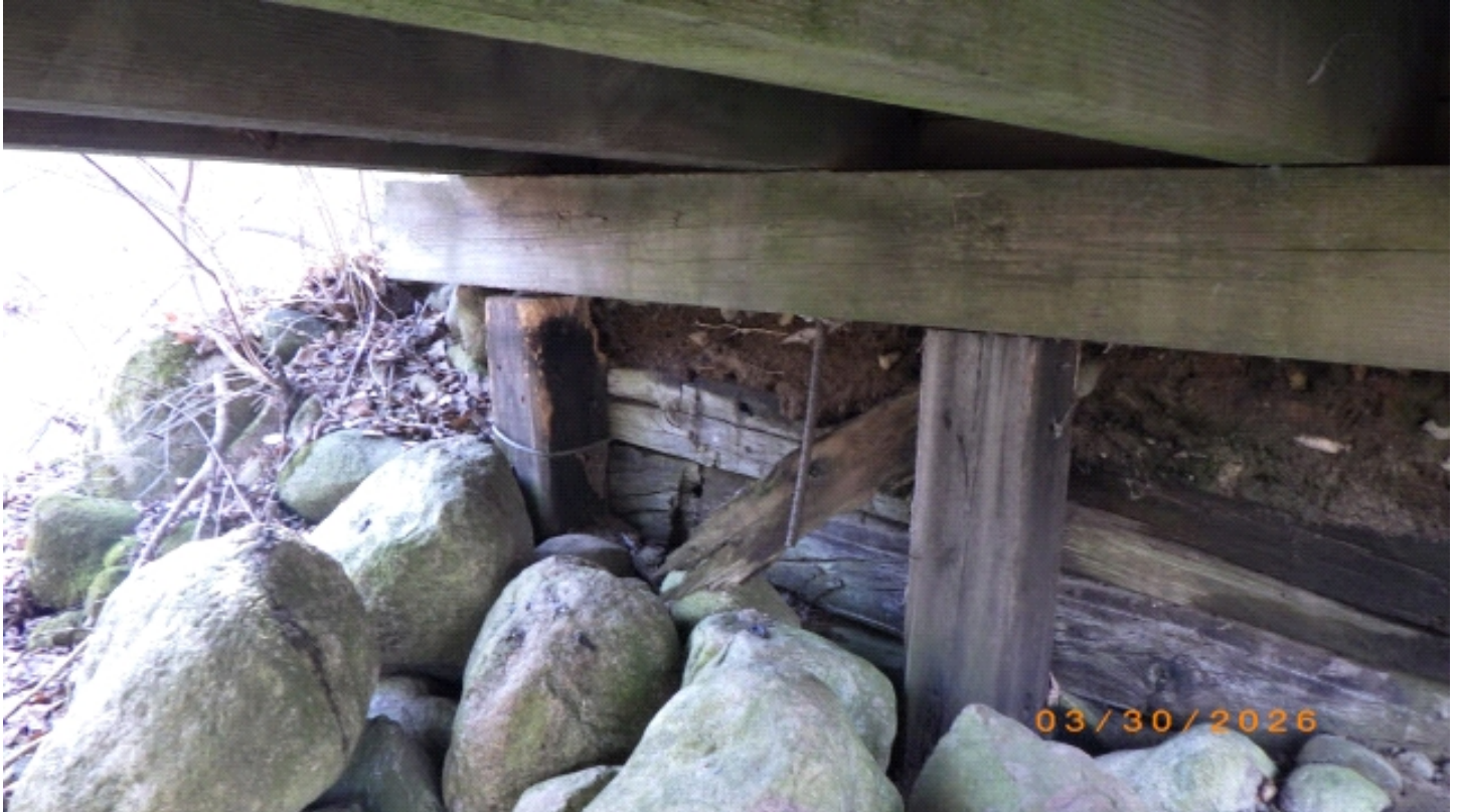
East end of South Abutment
