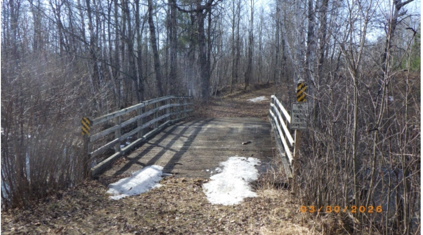
Looking South, Cut Brush Bad.
