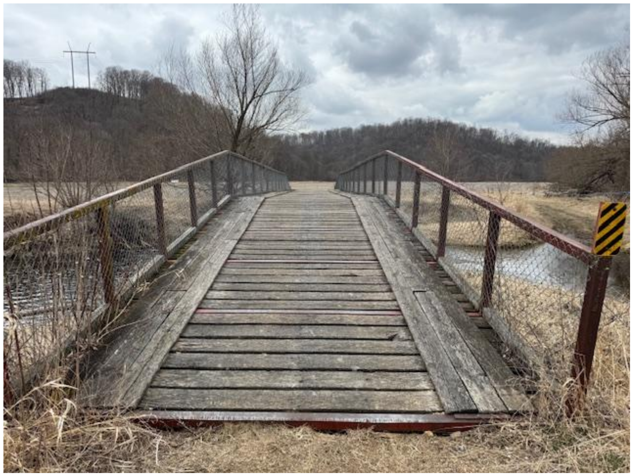
Approach from the south. Groomers are unable to cross this bridge and take a river crossing instead.
