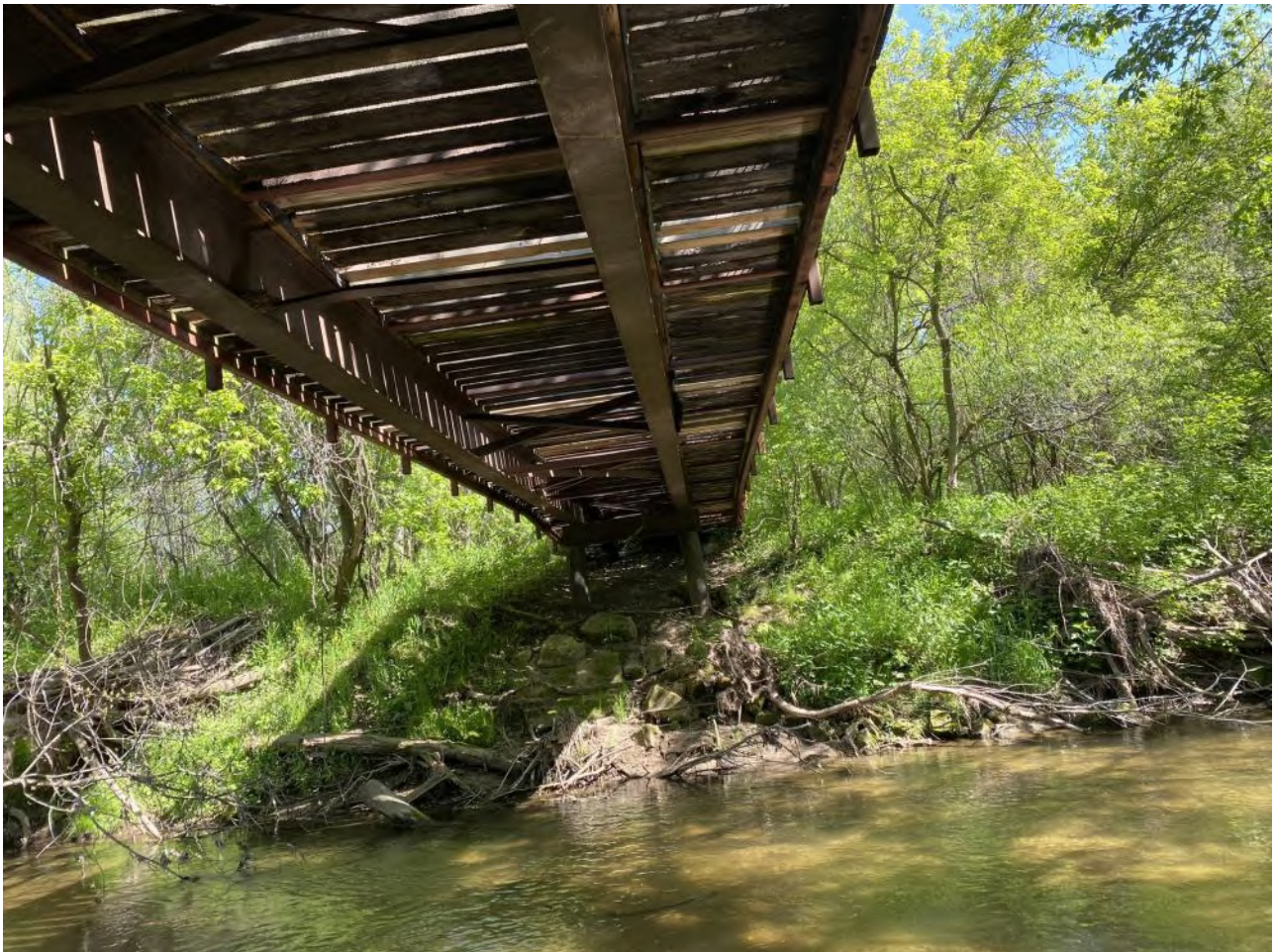
Narrow spaced I-Beam construction set on telephone poles
