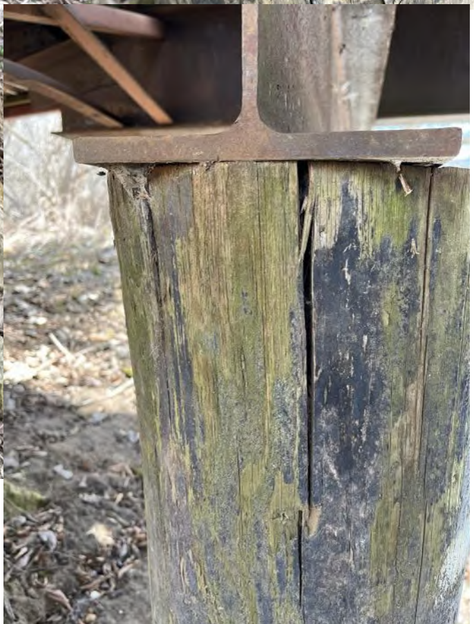
This is the worst post. Estimated to be mostly hollow with only 3" of good wood on the back side. The post is cracking pretty bad.
