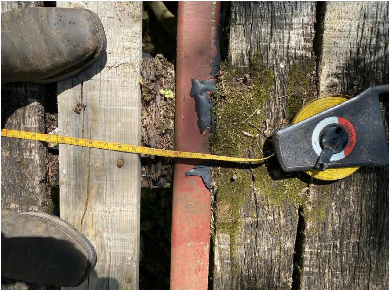
3x3 tubing is 6' apart. This may be the main thing holding up the tracked groomers.
