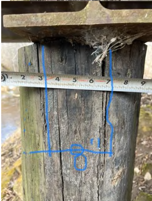
This is the worst post. Estimated to be mostly hollow with only 3" of good wood on the back side. The post is cracking pretty bad.
