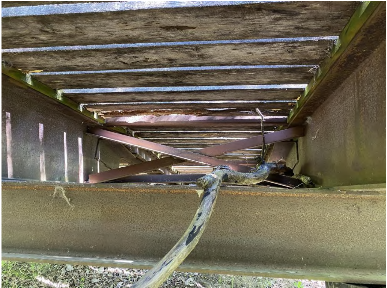
Ramp Attachment and crossmembers on inside
