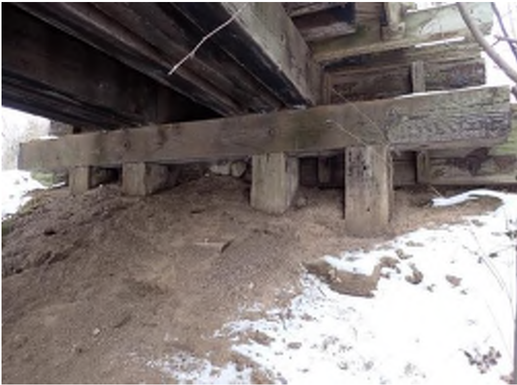
East abutment, looking northeast (taken Jan 2026)
