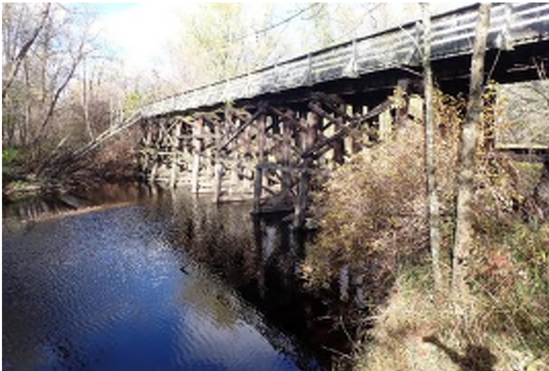
South fascia, looking northwest (taken Oct 2025)
