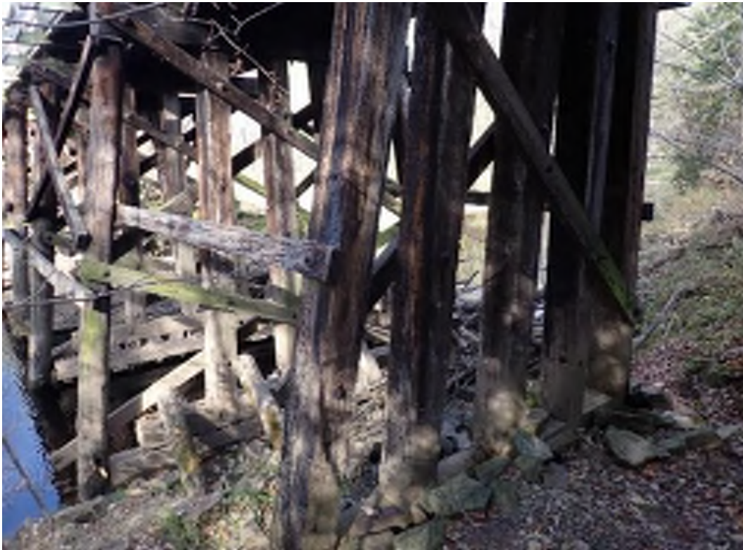
Typical pier and bracing, looking northwest (taken Oct 2025)
