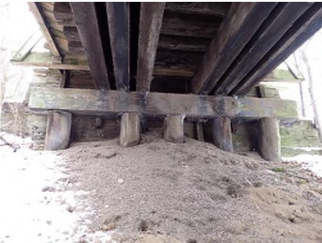
West abutment, looking west (taken Jan 2026)
