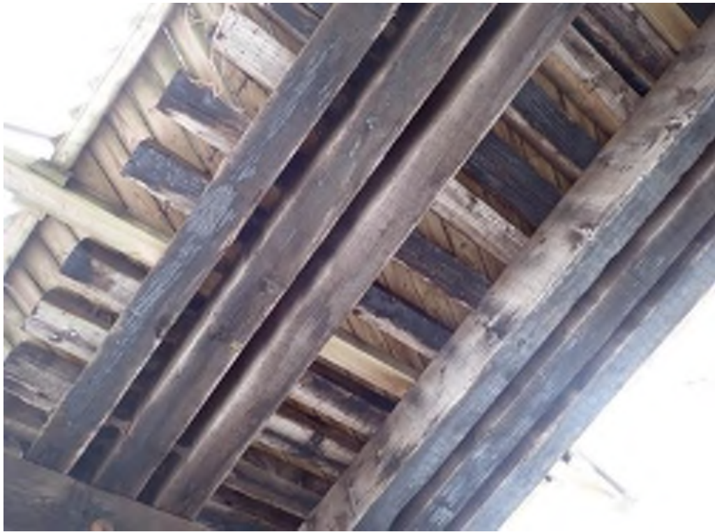
Typical underdeck, looking northwest (taken Jan 2026)
