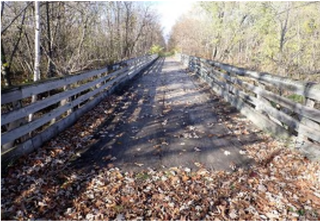
Overall view, looking west (taken Oct 2025)
