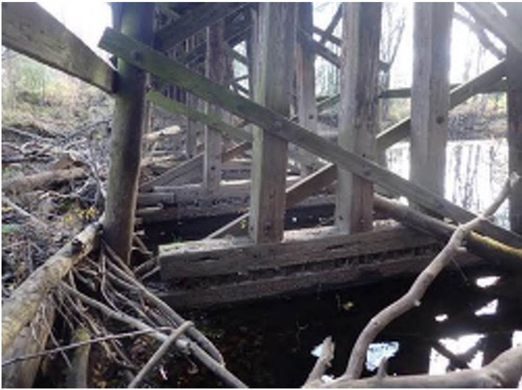
Typical pile cap, looking southeast (taken Oct 2025)
