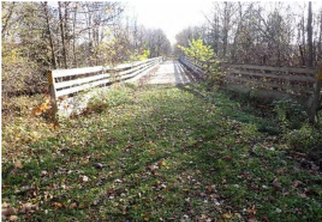
Overall view, looking east (taken Oct 2025)
