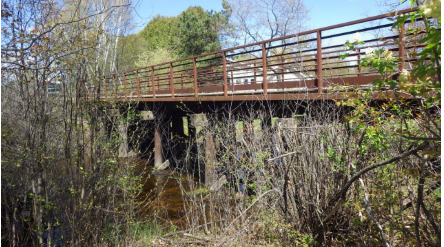
Upstream elevation view
