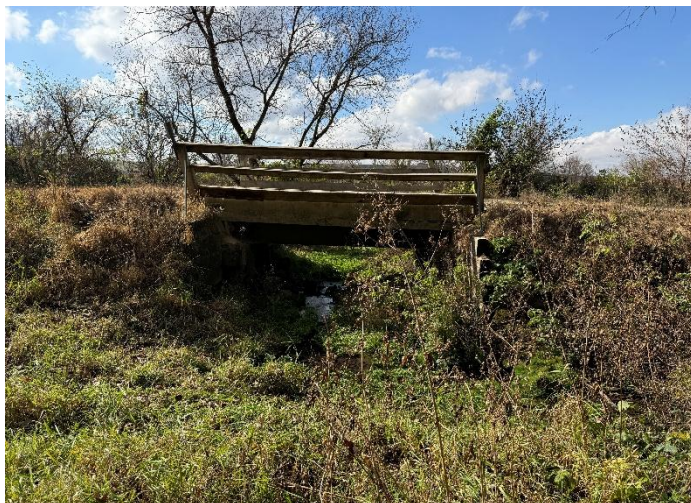
Photo 5 – Side View Looking West.
