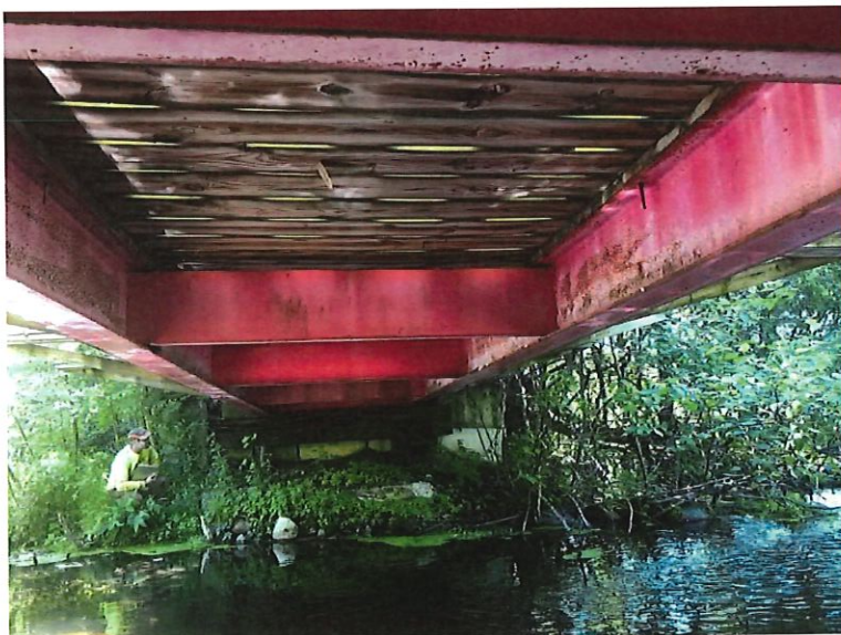
Bridge Substructure Looking West
