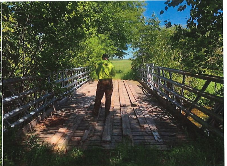
Bridge Deck Looking East
