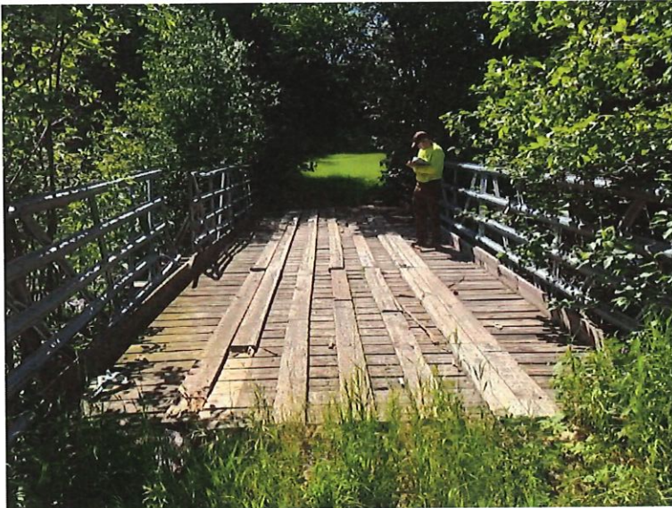
Bridge Deck Looking West
