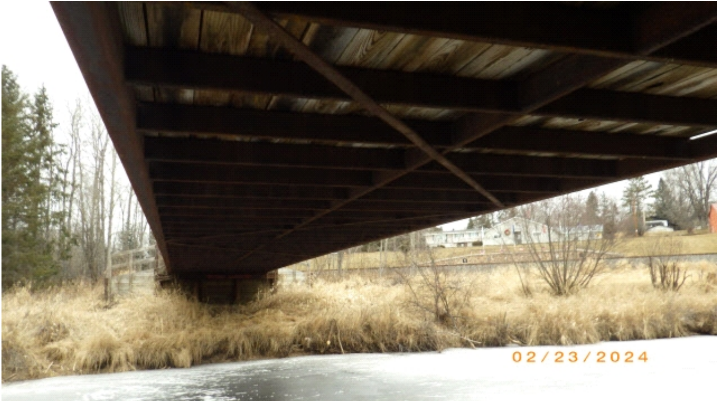
Bottom of deck, typical, looking West.
