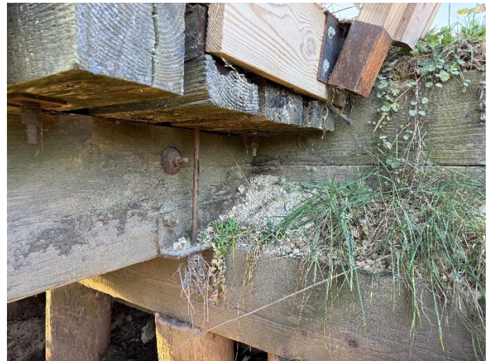
Photo 10 – West beam Over South Abutment.
