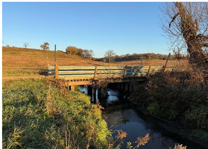
Photo 5 – Side View Looking West.
