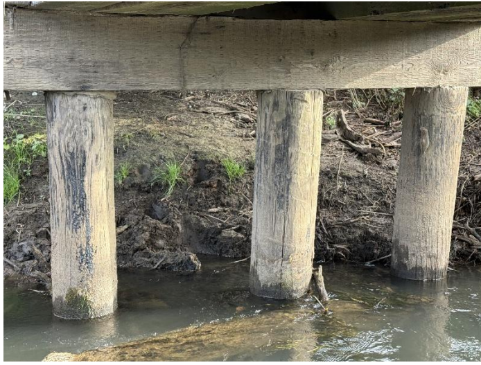
Photo 13 – North Pier Looking North: Piles W2-W4.
