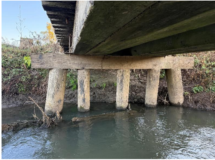
Photo 7 – North Pier Looking North.
