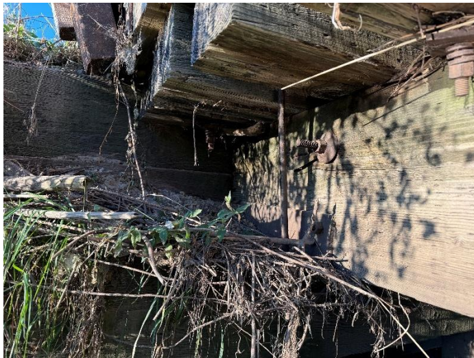
Photo 9 – East Beam Over South Abutment.
